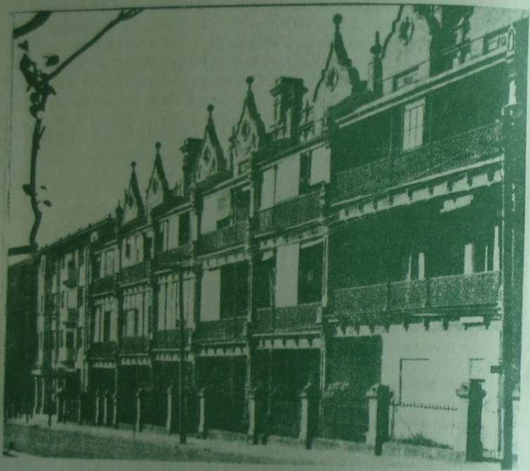
Before the green ban! People's homes, like these in Elizabeth Bay Road, Kings Cross, were demolished and the residents dispersed - to where?
