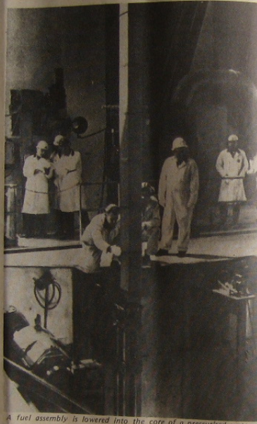
A fuel assembly is lowered into the core of a pressurised water reactor.
