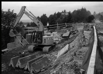
Sea to Sky highway construction, 2006
