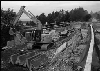
Sea to Sky highway construction, 2006
