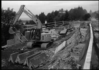
Sea to Sky highway construction, 2006
