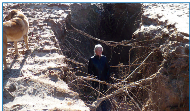
Eleanor Fairchild stands in an erosion area adjacent to a wetland after pipeline construction on her property.
