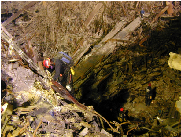
Fig. 19 - Liberty St. Hole #2, next to basement of WTC 2 (Sept. 18)
