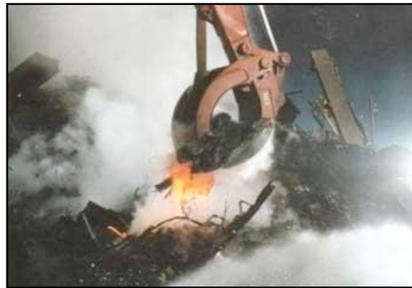
Fig. 18 - An excavating machine at Ground Zero lifts debris dripping with molten metal
