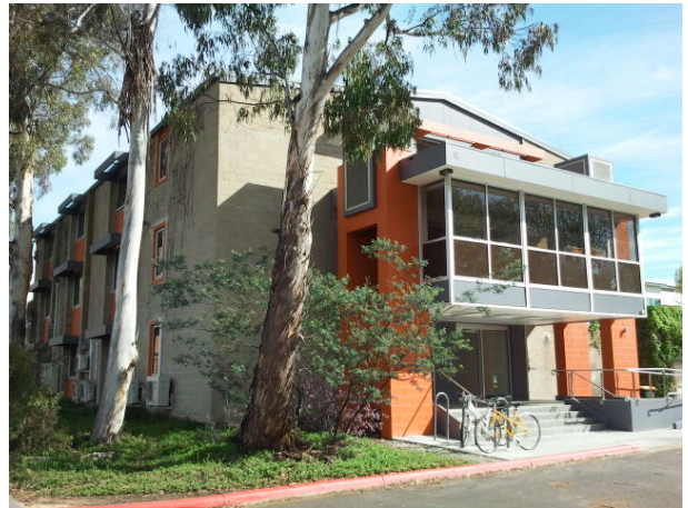
John Yencken Building, 45 Sullivans Creek Road, ANU campus.
