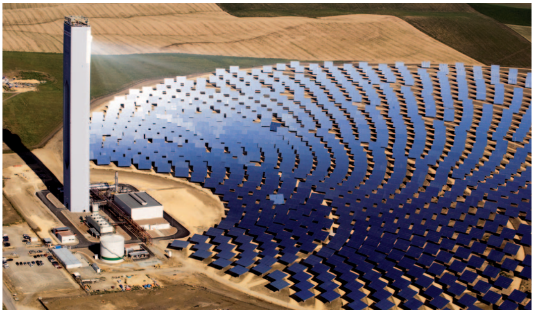
PS20 concentrating solar thermal power tower near Sevilla, Spain.
