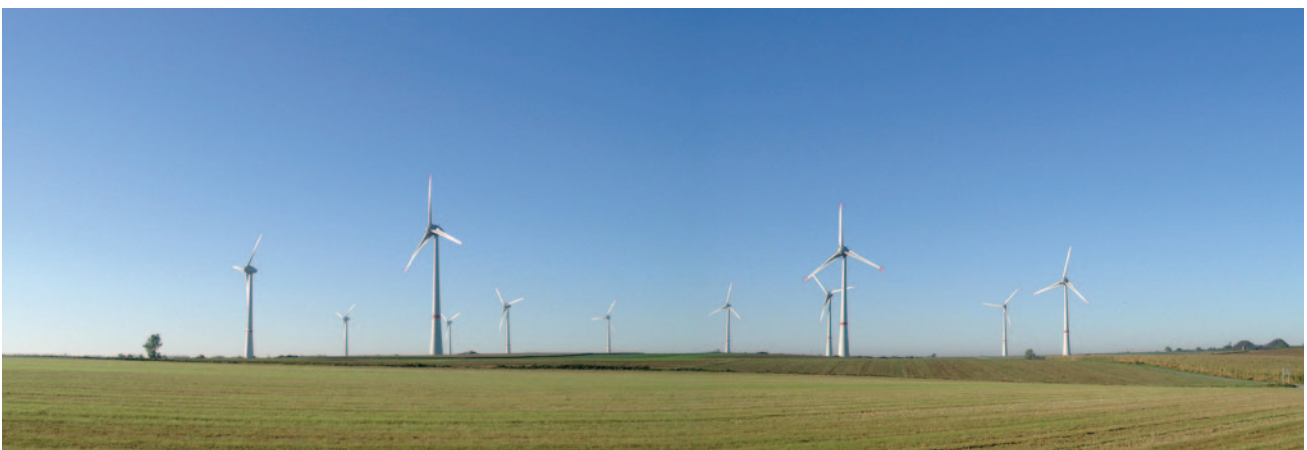
Enercon 7.5MW permanent magnet direct-drive wind turbines in operation, Estinnes Wind Park, Belgium.
