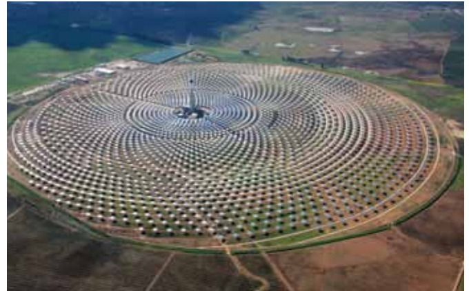
Figure 5: Torresol Gemasolar plant Spain, courtesy Torresol
