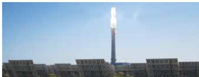
Above: Heliostat mirrors and central tower receiver at the Torresol Gemasolar power plant, Spain. Image courtesy of Markel Rodondo.
