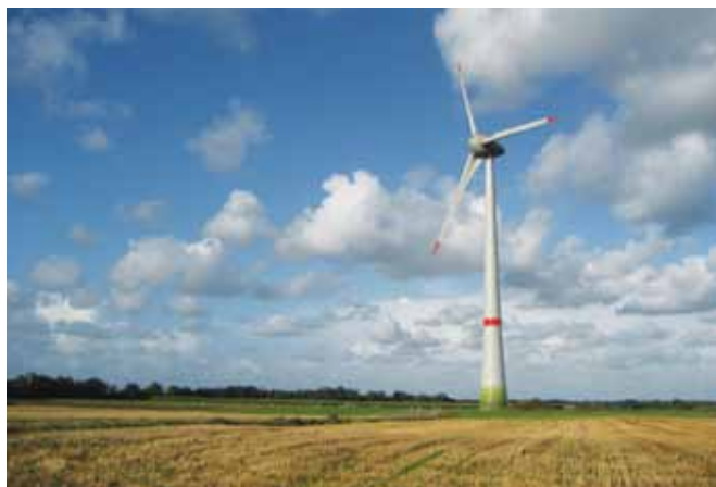
Above: Enercon E126 7.5 MW wind turbines at Estinnes, Belgium. Courtesy Enercon
