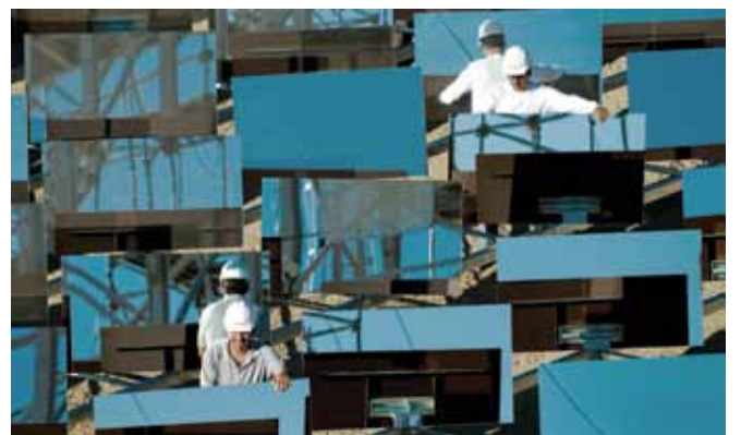
Above: Heliostat mirrors being installed at Esolar plant California
