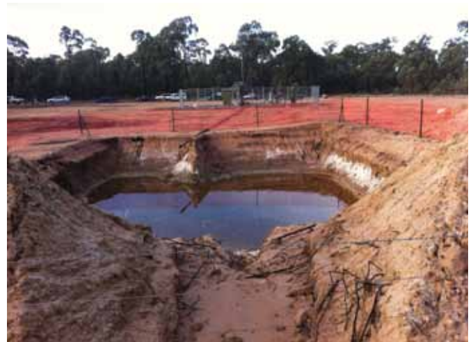
Above: Santos operated coal seam gas well, Pilliga State Forest, New South Wales.
