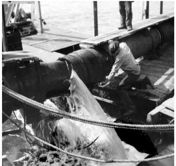
Pontoons and Dredging Pipe - (Courtesy of San Francisco History Center, San Francisco Public Library)
