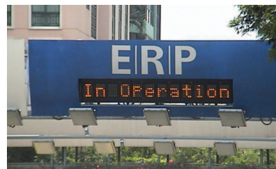
FIG5 Singapore's electronic road pricing (ERP) using RFID was launched by the Singapore Land Transport Authority in 1998. It was the world's first ERP system, an automated toll-collection system used to control and manage traffic volume in the city. (Photo courtesy of Katina Michael.)
