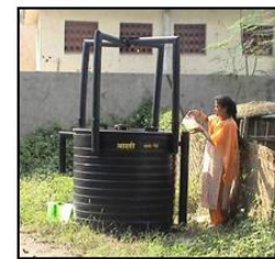
India: household biogas System
