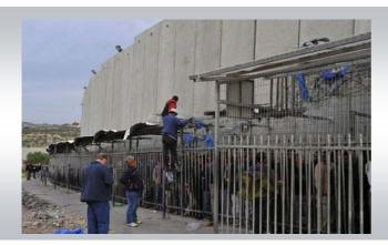
The Wall is comprised of 8-metre high concrete walls, ditches, trenches, electric-fences, patrol roads and barbed wire. As currently projected, the Wall will be 725 km long when complete.
