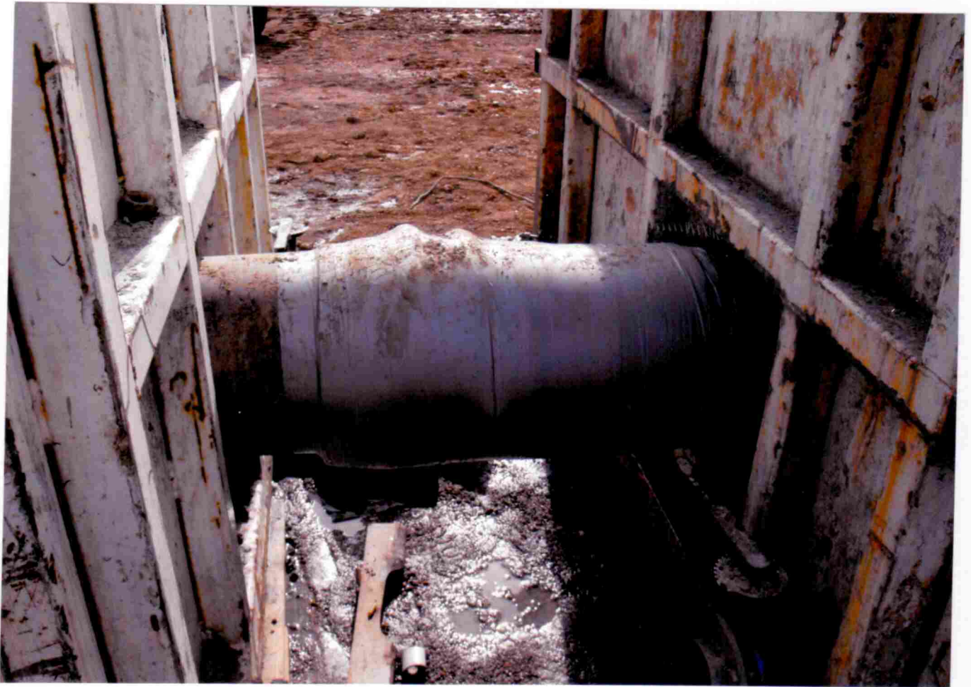
7. and 8. Contaminated Water Storage Tanks joined showing leakage of High Saline Water on to Ground
