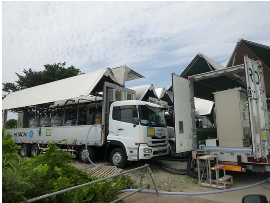
credit: Tokyo Electric Power Company photo: August 13, 2014
