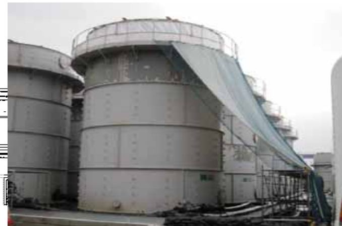
Completion of installation of protection tent for countermeasure testing
