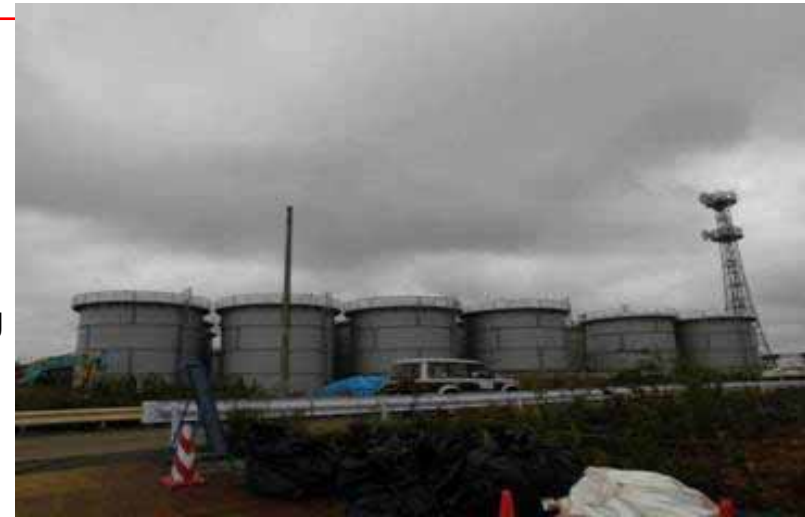
Full view of the east side of the H4 area
