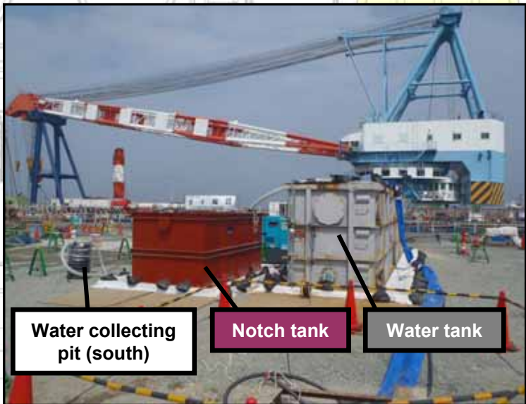
Photo taken by TEPCO on August 9, 2013
