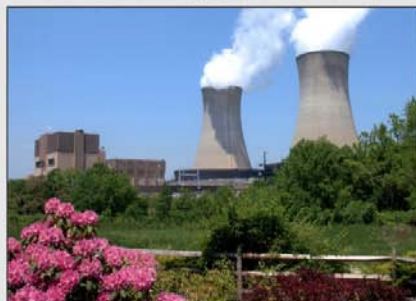
Limerick Generating Station – Limerick, PA
