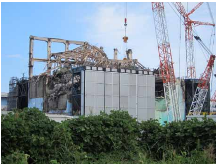
-3 Upper part of Unit 3 Reactor Building
