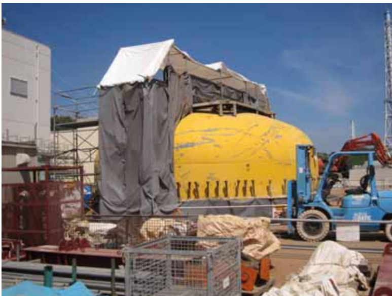
-2 Unit 4 PCV lid being cut off
