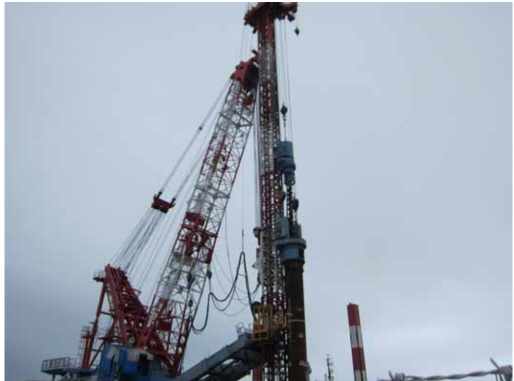
Impermeable wall piling ship
