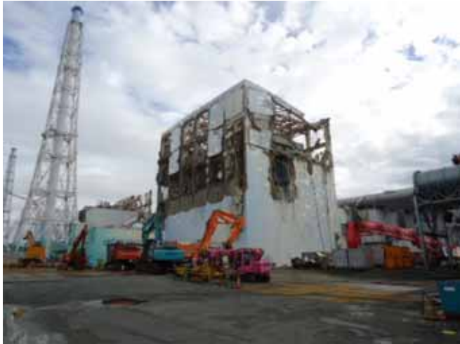
-1 Debris removal from the upper part of Unit 4 Reactor Building (Before removal)
