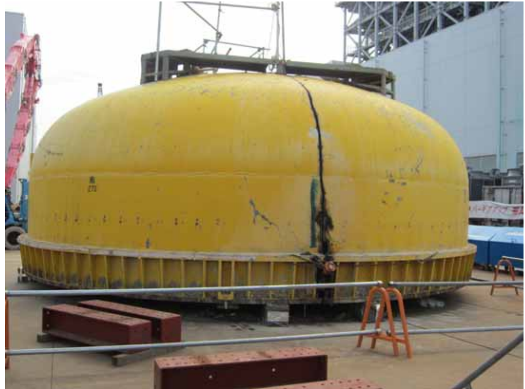
-3 Unit 4 PCV lid (After being cut off)
