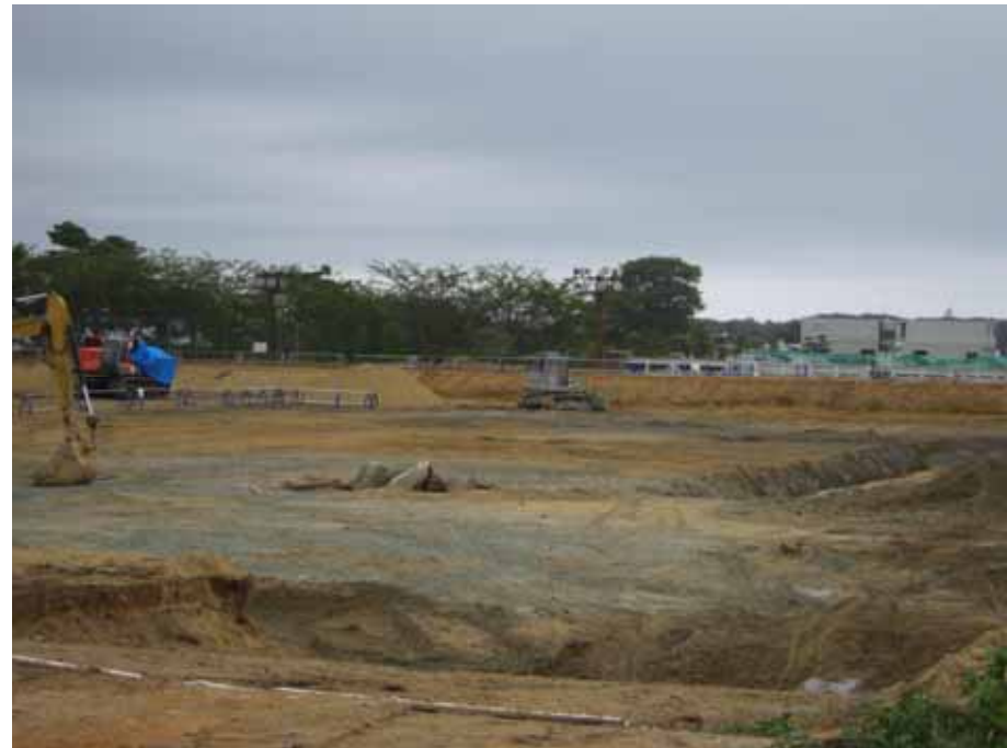
Land development for the dry cask temporary storage facility
