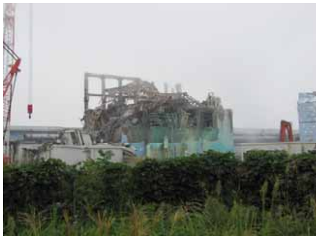
-1 Upper part of Unit 3 Reactor Building (Before the debris was removed)
