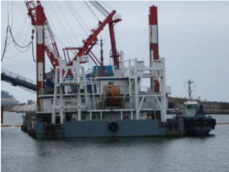
Impermeable wall piling ship
