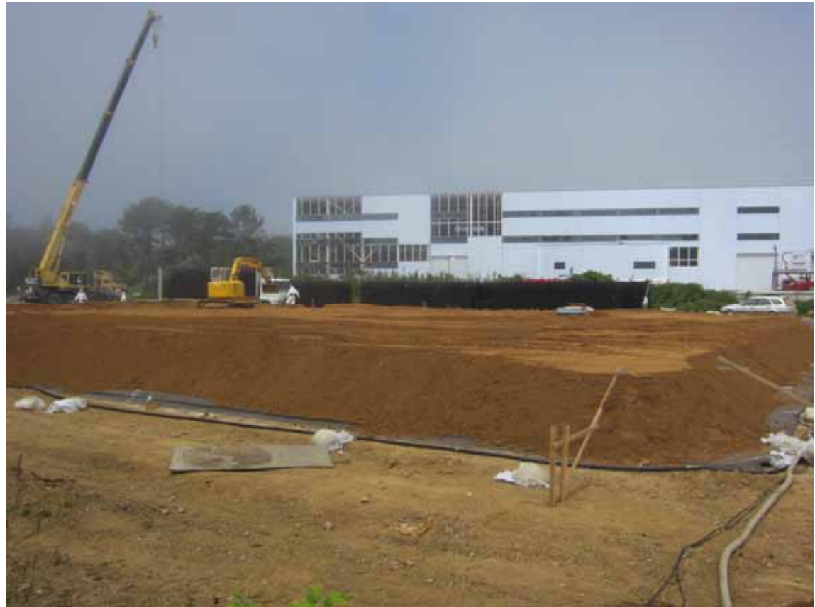
-2 Underground water storage tank installation
