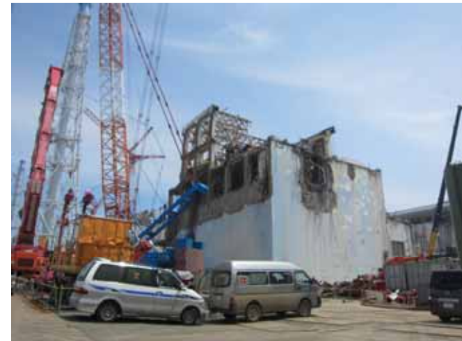
-3 Unit 4 Reactor Building
