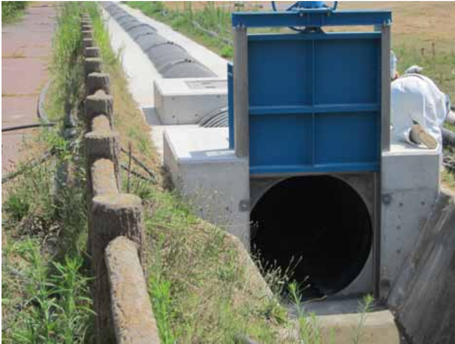
Drainage (polyethylene pipe) installation in the power station site
