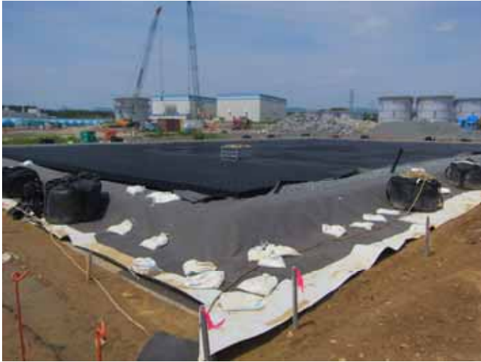
-1 Underground water storage tank installation
