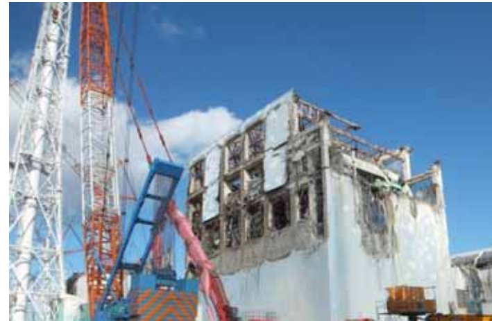
-2 Debris removal from the upper part of Unit 4 Reactor Building (During removal)
