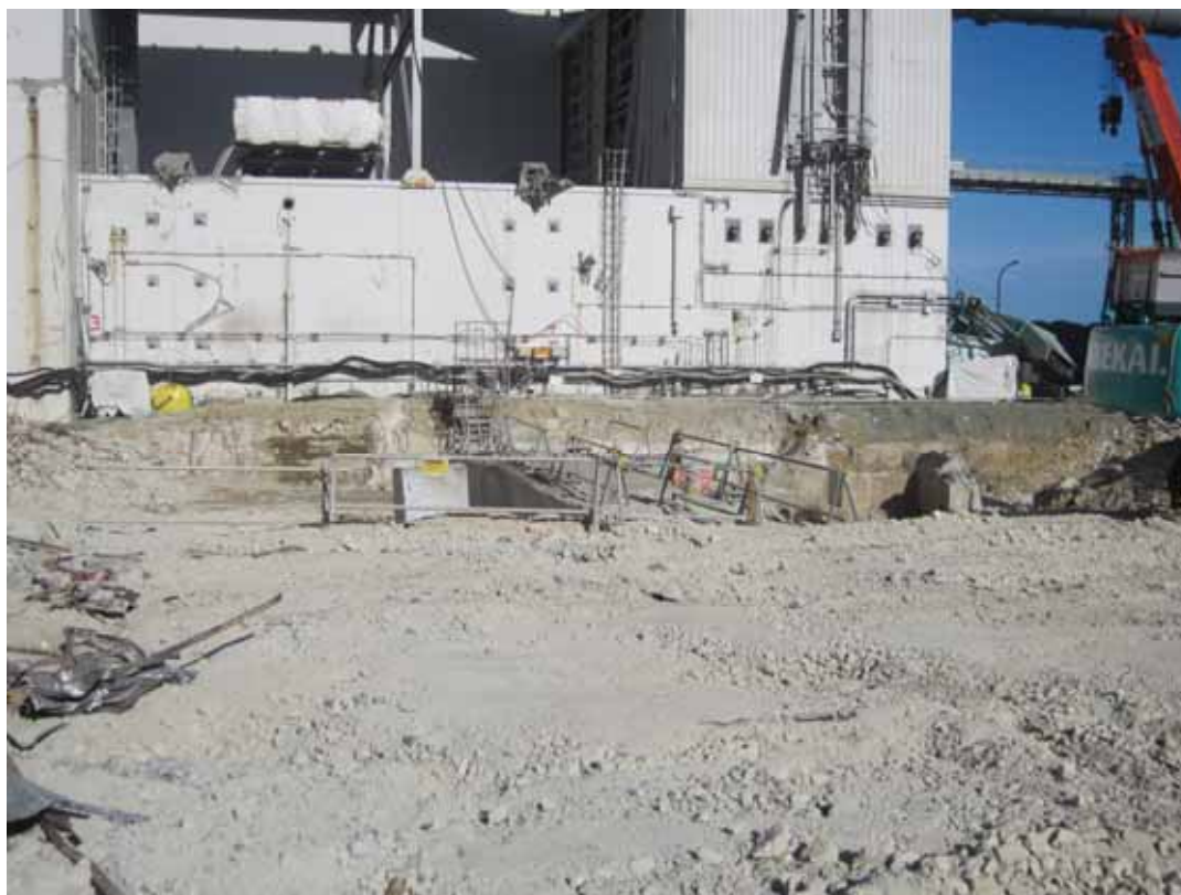
-2 Unit 4 south side foundation improvement work (After completion)
