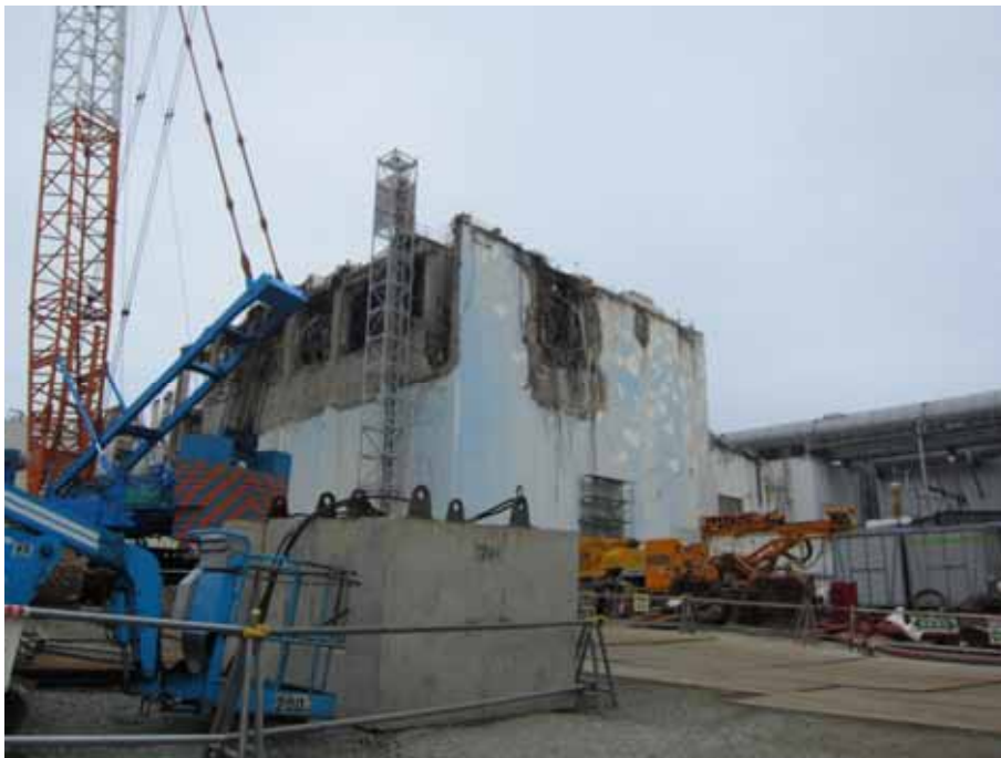
-4 Unit 4 Reactor Building
