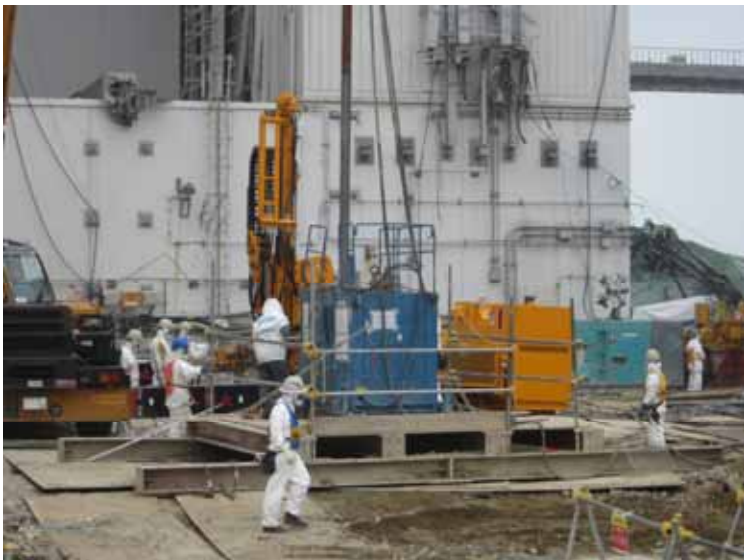
-1 Unit 4 south side foundation improvement work: Foundation improvement equipment
