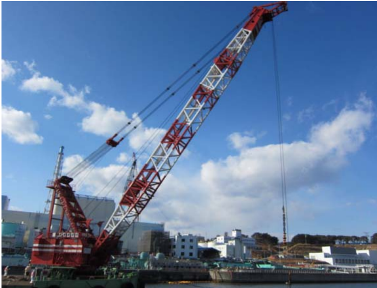
③-4 Removal of obstacle by the floating crane (from east breakwater)
