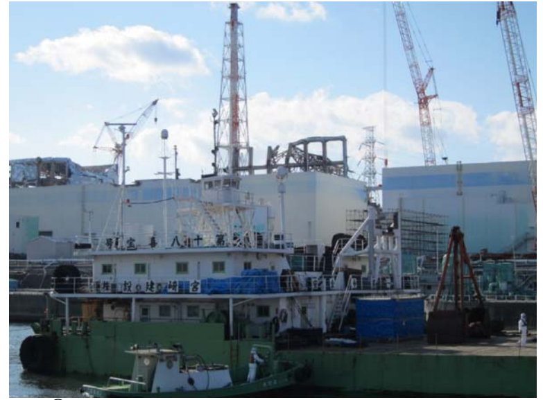
③-5 Removal of obstacle by the floating crane (from east breakwater)
