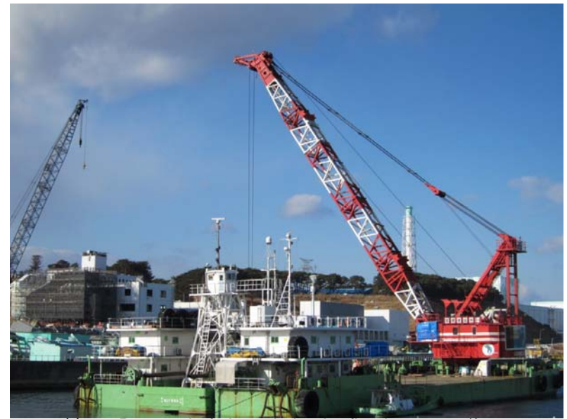
③— 2 Removal of obstacle by the floating crane (from east breakwater)
