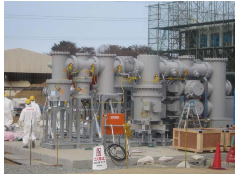
⑦-6 Construction of new switch station Jan. 9, 2011 photo by TEPCO staff
