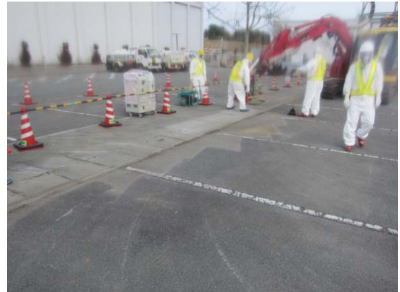
②-9 Collection work of dust and small debris at parking area of Main Anti-earthquake Building (after work)
