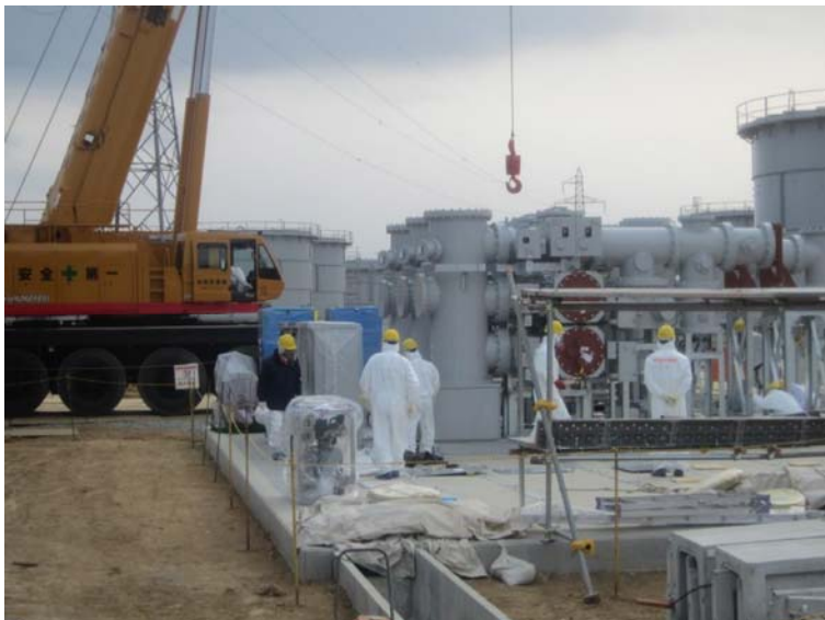
⑦-3 Construction of new switch station Jan. 9, 2011 photo by TEPCO staff
