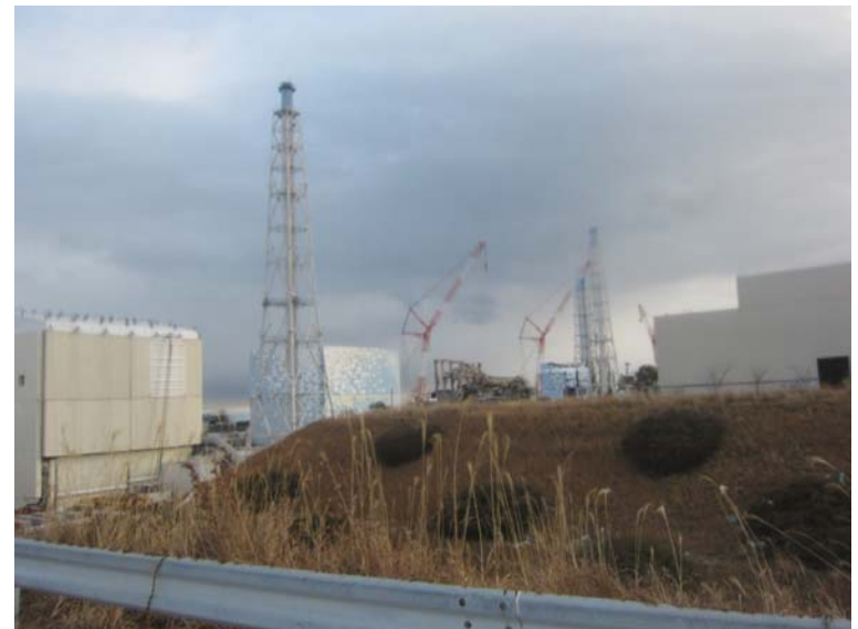
⑪-4 Look into Unit 2,3 Reactor Building from the backside of Main Anti-earthquake Building
