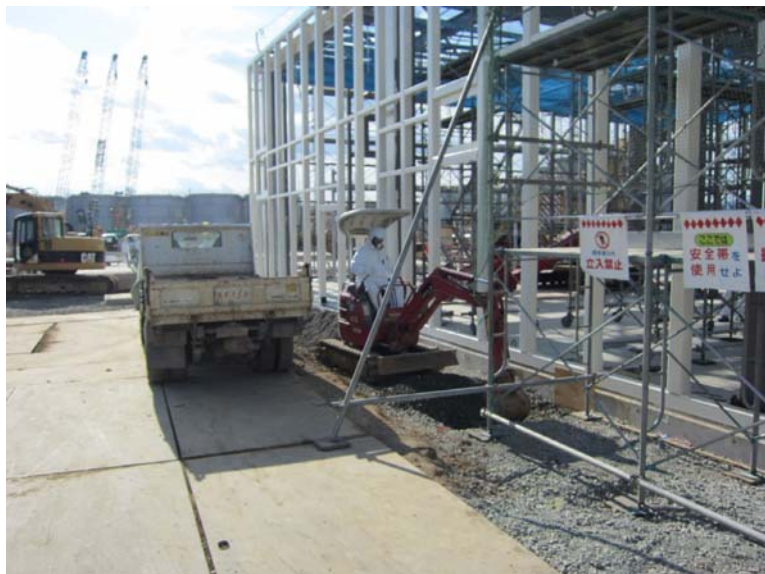
⑦-8 Construction of new switch station Jan.10, 2011 photo by TEPCO staff
