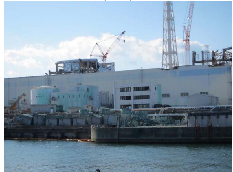
③— 3 Unit 3,4 Turbine Building (from east breakwater)
