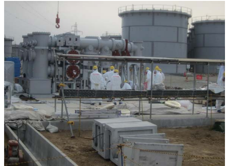
⑦-2 Construction of new switch station Jan. 9, 2011 photo by TEPCO staff
