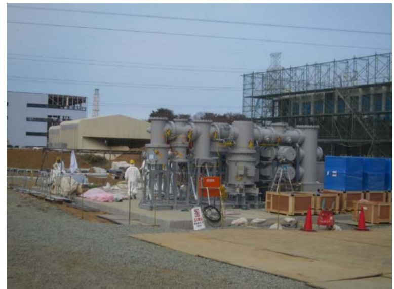
⑦-7 Construction of new switch station Jan. 9, 2011 photo by TEPCO staff
