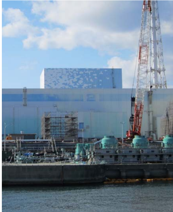
③— 1 Unit 2 Turbine Building (from east breakwater)
