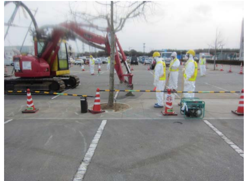
②—5 Collection work of dust and small debris at parking area of Main Anti-earthquake Building
