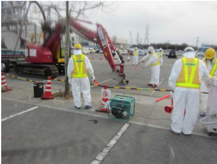
②—4 Collection work of dust and small debris at parking area of Main Anti-earthquake Building
