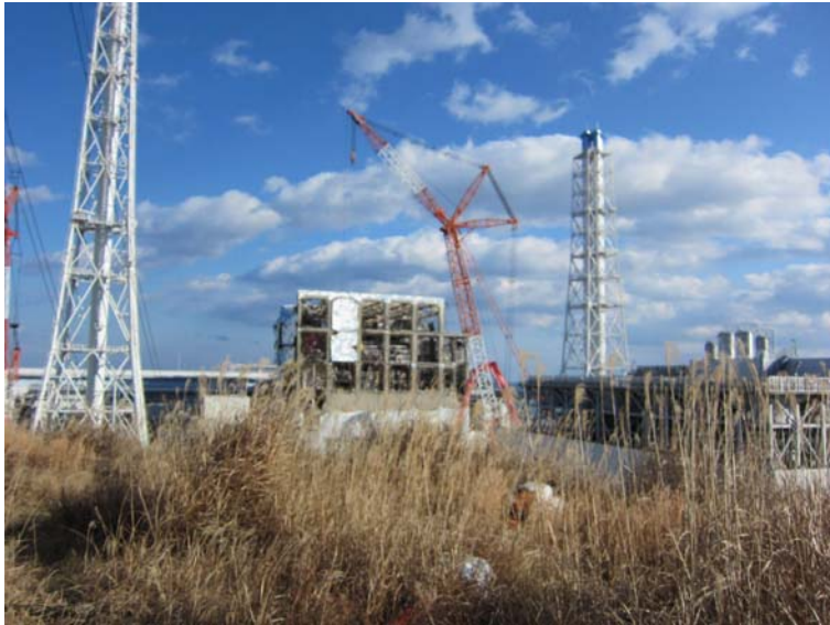
⑭— 1 Unit 4 Reactor Building Jan. 14, 2012 photo by TEPCO staff
