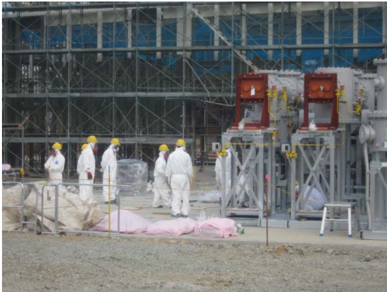
⑦-5 Construction of new switch station Jan. 9, 2011 photo by TEPCO staff
