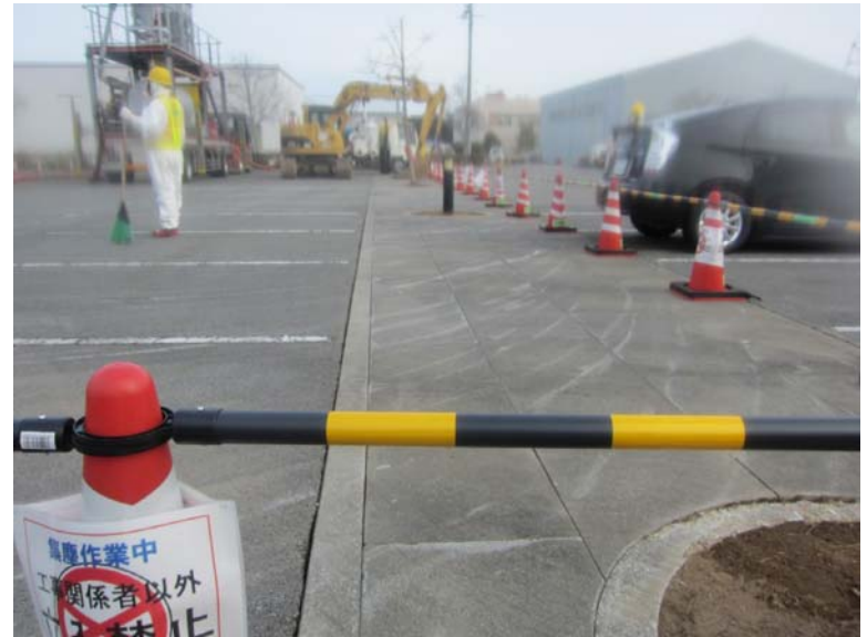
②-8 Collection work of dust and small debris at parking area of Main Anti-earthquake Building (after work)
