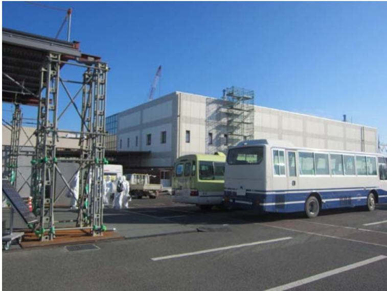
⑤ Main Anti-earthquake Building Jan. 18, 2012 photo by TEPCO staff
