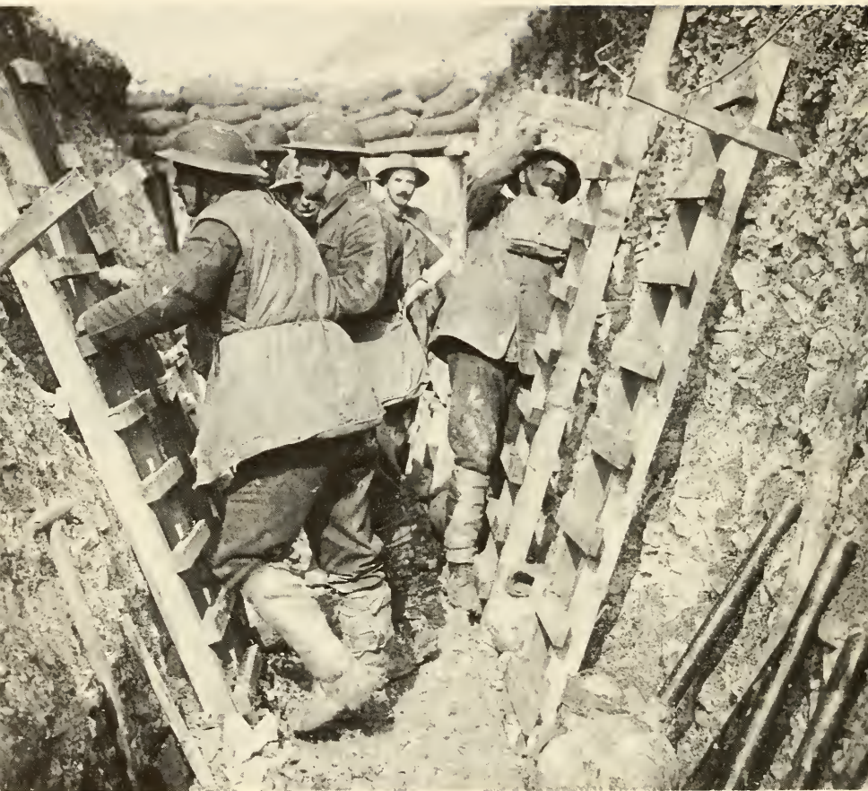
Scaling ladders are positioned in anticipation of a forthcoming assault.
