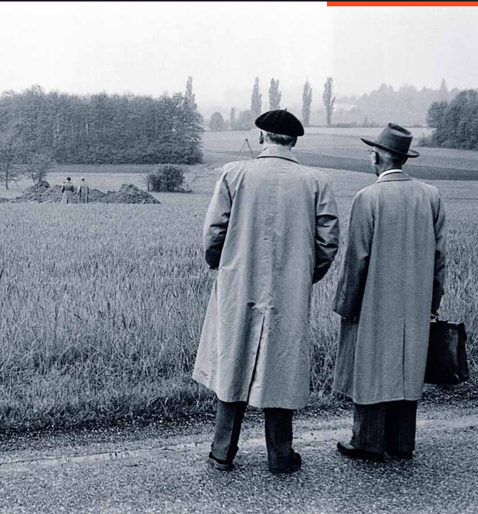
2. Construction officially begins on the Meyrin site in Switzerland on May 17th, 1954.
