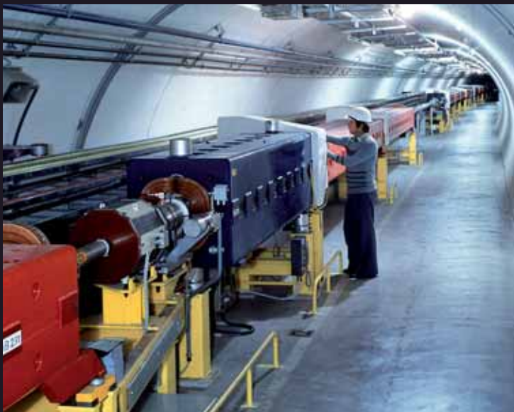
8. 9. Completed in 1976, the 7 km-long Super Proton Synchrotron (SPS) was the first giant underground ring to cross the Franco-Swiss border. Today, it accelerates particles before feeding them to the Large Hadron Collider (LHC); a 27 km ring buried 100 m below ground, housing two high-energy particle beams travelling in opposite directions.
