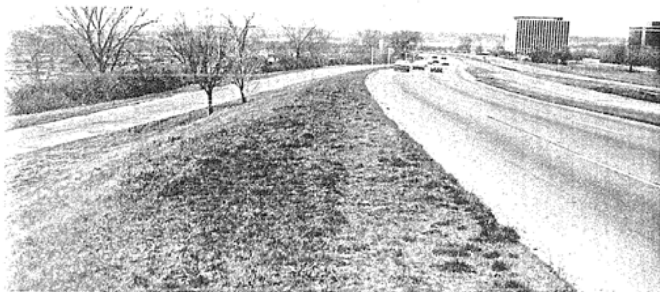
Shirley Highway, facing east. The ramp on the left is an access to Washington Blvd., "South", which leads to Arlington Naval Barracks and Henderson Hall of the US Marine Corps headquarters. Directly to the left is the Pentagon South Parking Area. In the background, the Potomac River can be seen.
