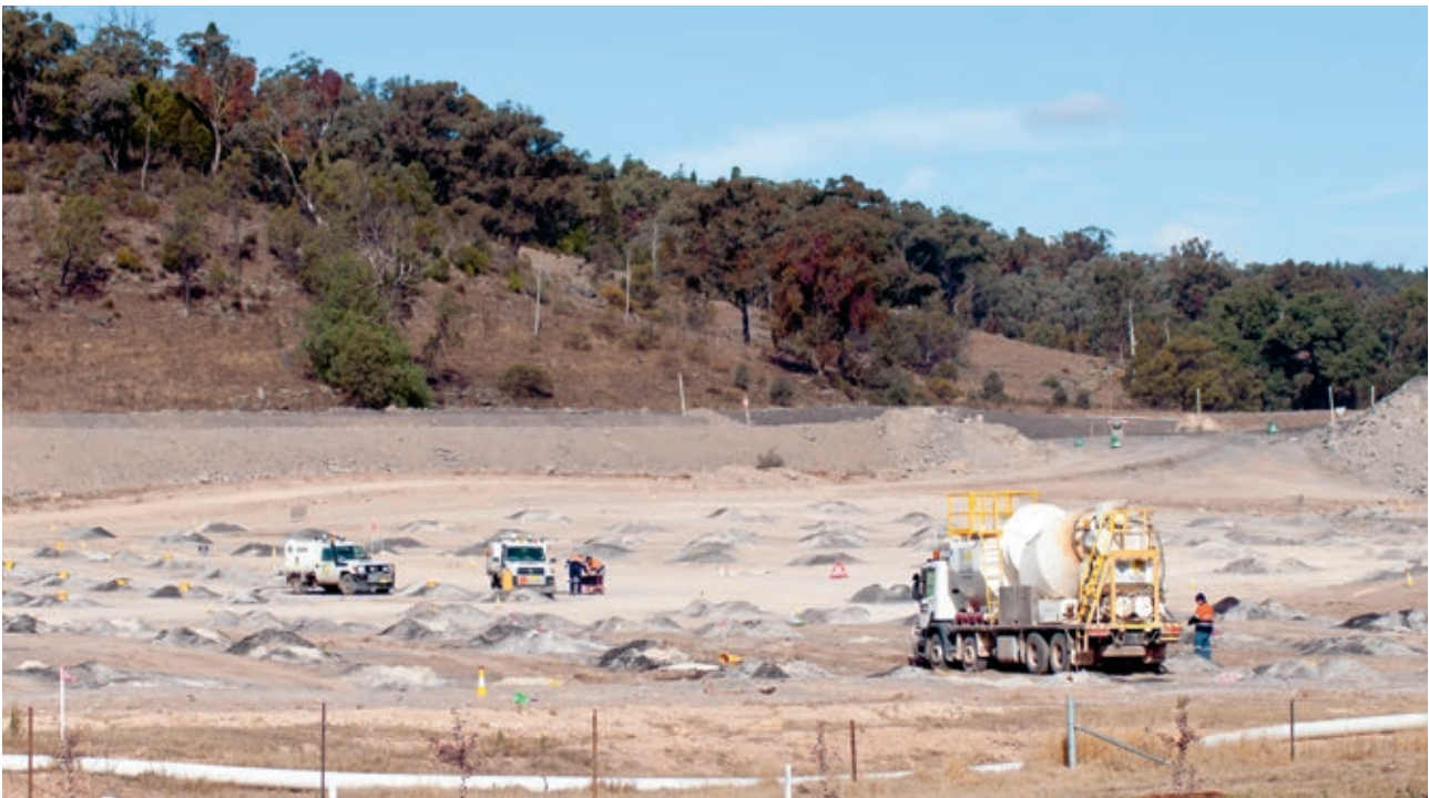
Laying explosives at Moolarben. Photo: Max Phillips
