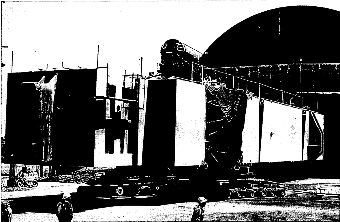
Figure 21. Strongback being loaded on the HMB-1 at the Ambridge plant in South San Francisco
