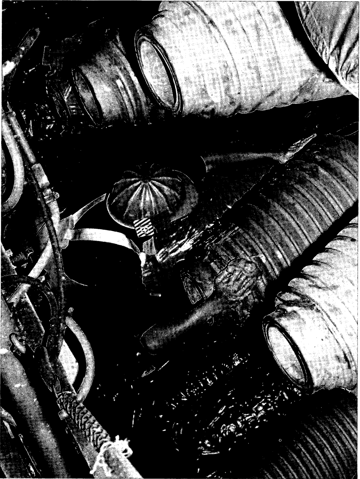
Figure 31. Applying Aqua-Lube to the threads. It didn't work and had to be removed.
