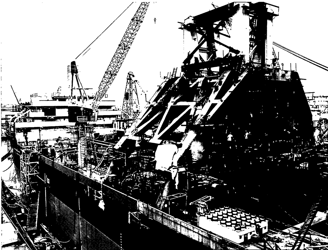
Figure 11. A-frame structure which provided the load path from the lift system to the ship
