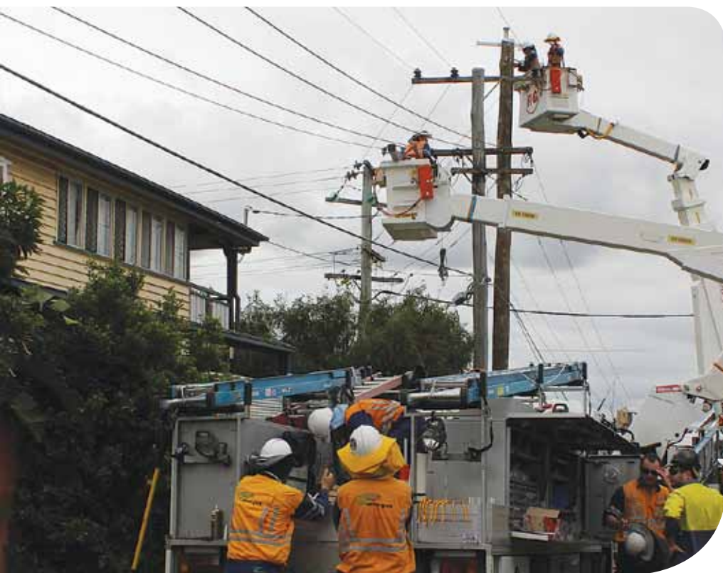
The importance of safety – Energex overhead crews at work.
