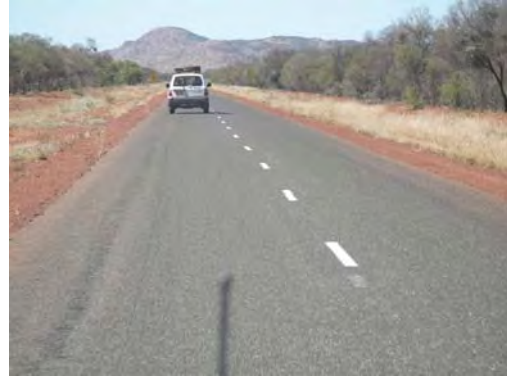
PHOTOGRAPH T3.4 Tanami Road – short widened section
