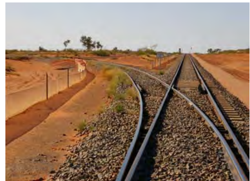
PHOTOGRAPH T3.30 Rail turnout from mainline into Bootu Creek siding
