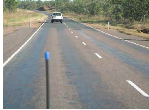
PHOTOGRAPH T3.18 Stuart Highway south of Katherine
