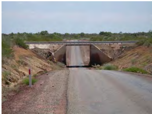
PHOTOGRAPH T3.24 Bootu Creek Mine haul road at Stuart Highway underpass
