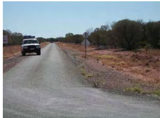
PHOTOGRAPH T3.5 Sealed access road to secure compound
