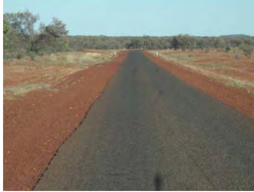
PHOTOGRAPH T3.3 Tanami Road west of Stuart Highway – typical standard
