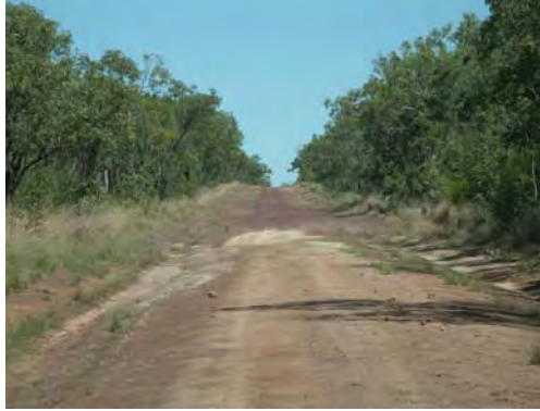
PHOTOGRAPH T3.20 Access road through site – view 1
