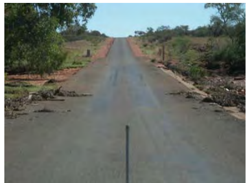
PHOTOGRAPH T3.11 Plenty Highway – typical floodway
