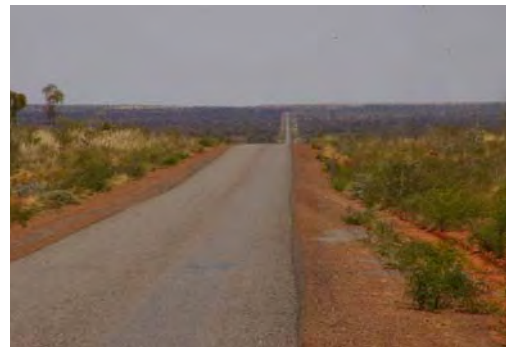
PHOTOGRAPH T3.25 Bootu Creek Mine haul road near repository site
