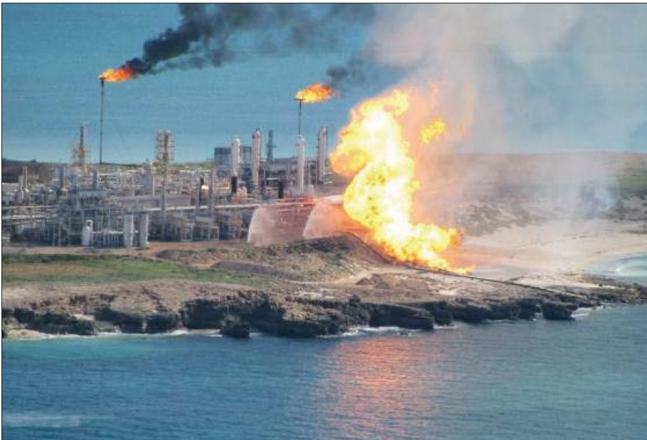
Photo 2 - Varanus Island fire and explosion incident, view from helicopter
