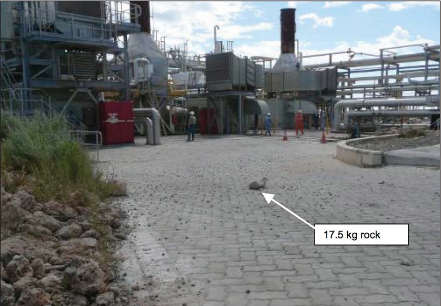
Photo 12 – Debris in HJV gas plant (compressors) area
