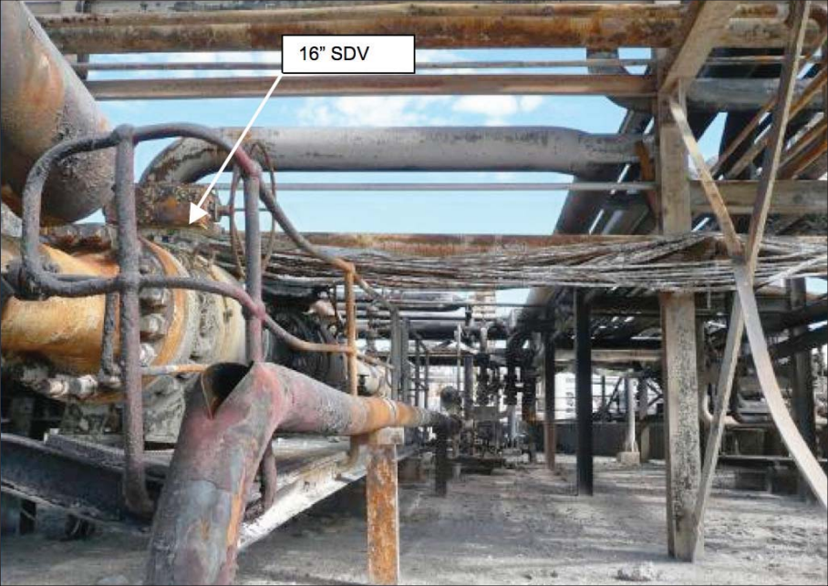
Photo 11 – Ruptured 6” Harriet gas line
