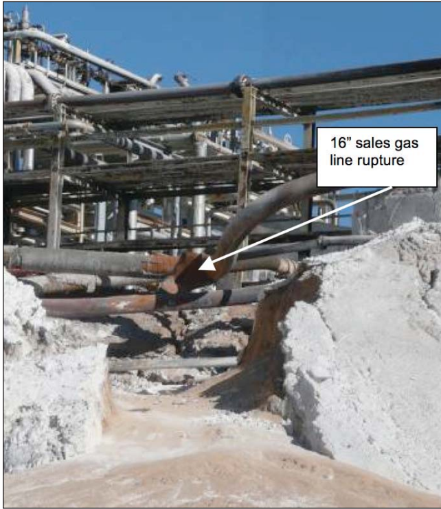
Photo 13 – Seawall banking water and jet fire erosion
