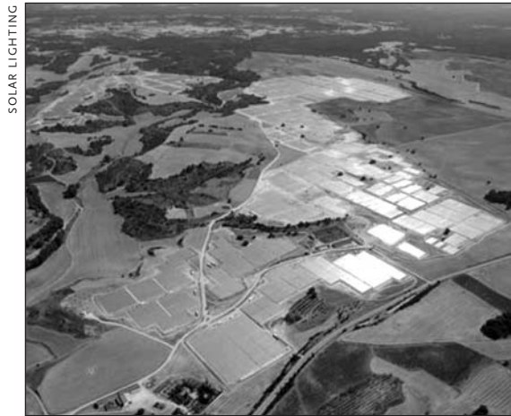
The 162,000 solar panels at Spain's 62 MW Olmedilla Solar Park (the world's largest photovoltaic power station) produce about 87.5 gigawatt-hours of electricity a year—enough to power more than 40,000 homes. The Olmedilla plant was constructed in just 15 months at a cost of $350 million.
