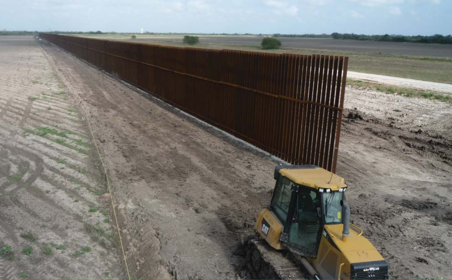
Construction of the US-Mexico border fence
