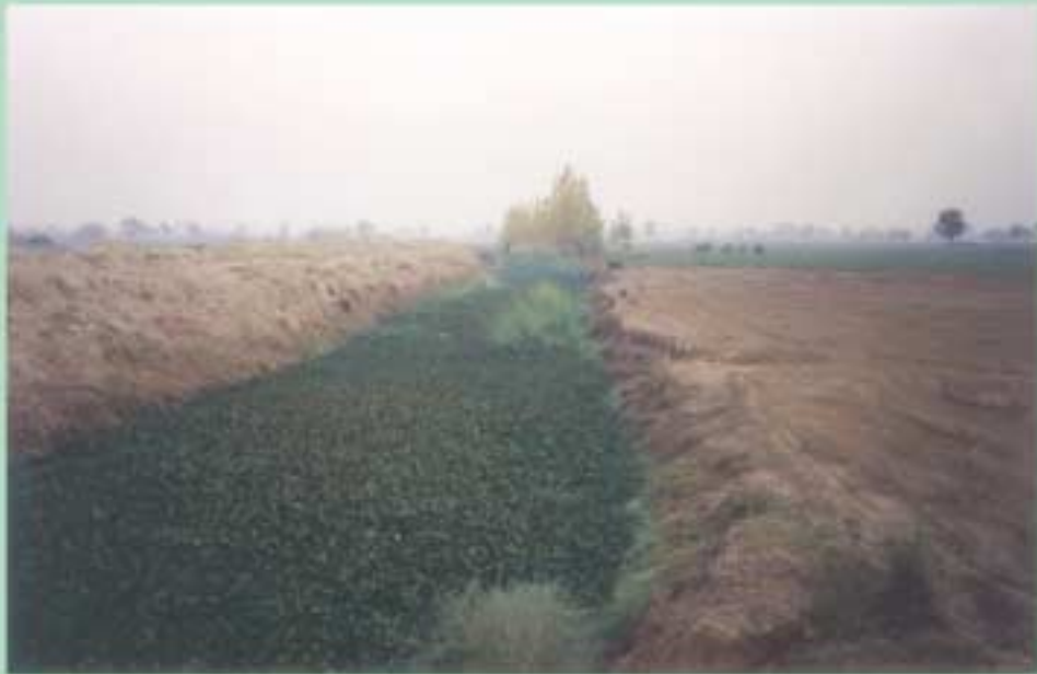
A drain nallah to control waterlogging, just outside Malout town, district Muktsar, Punjab. The nallah is choked with overgrowth of hyacinth. In places, the nallah is also used for disposal of sewage, effluents etc.
