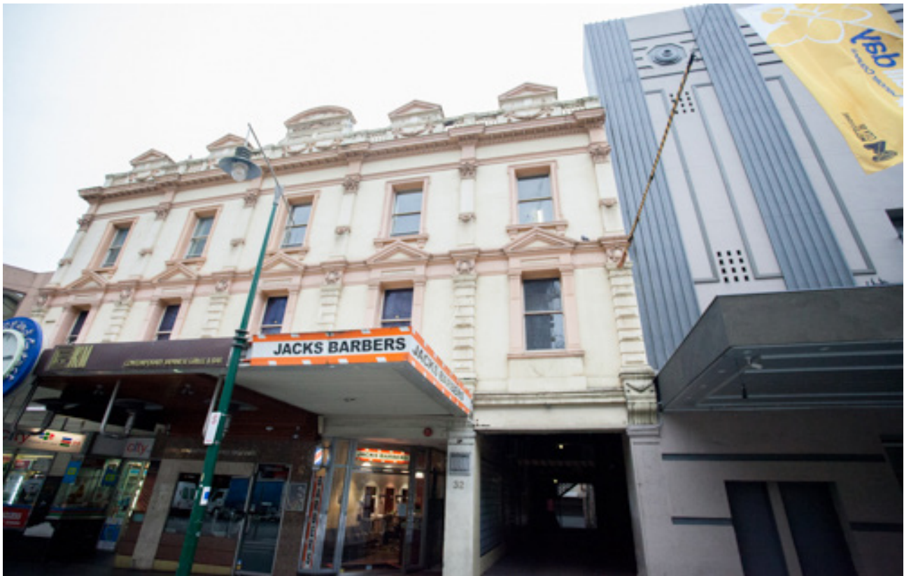
The intact row of 1892 terraces, next to the Art Deco facade of the Palace
