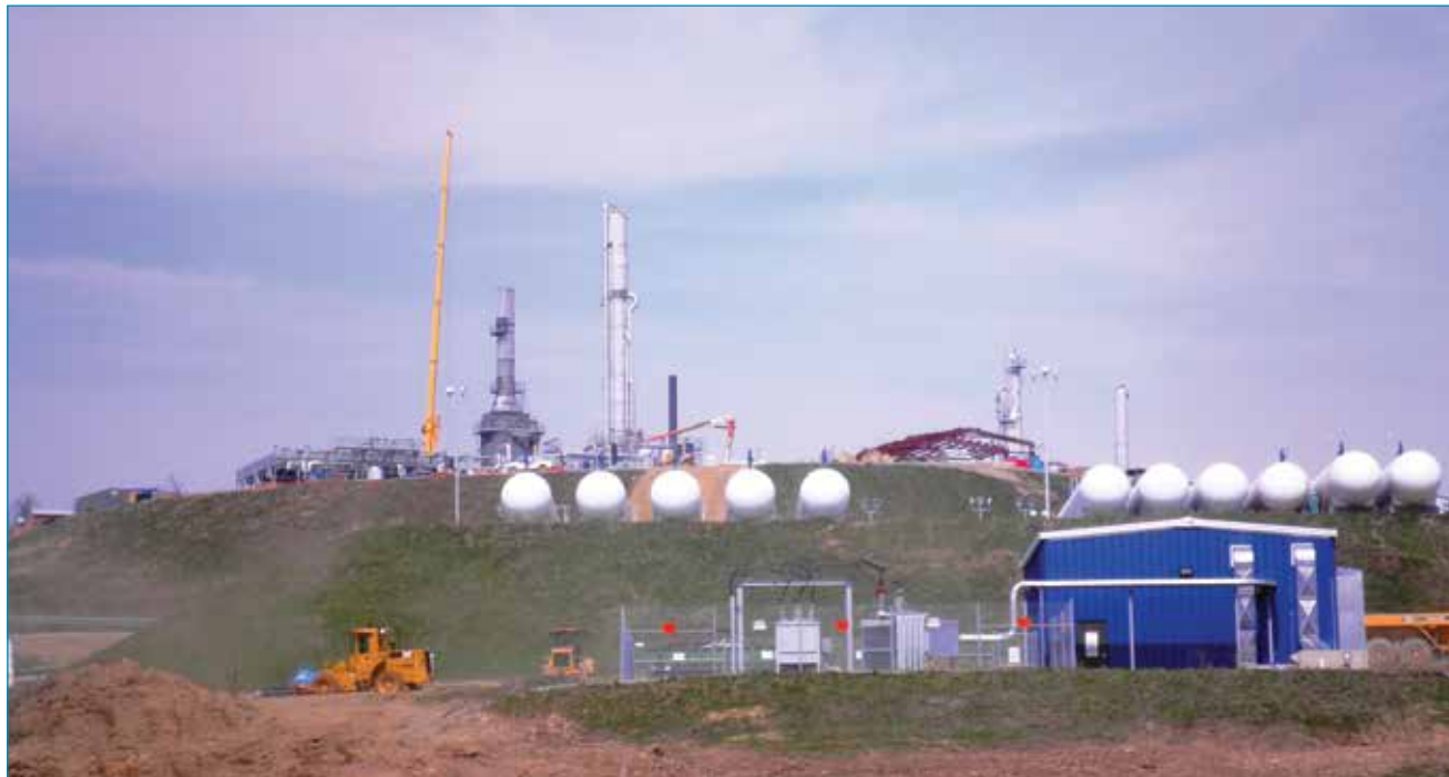
Gas processing plant near Houston, Pennsylvania
