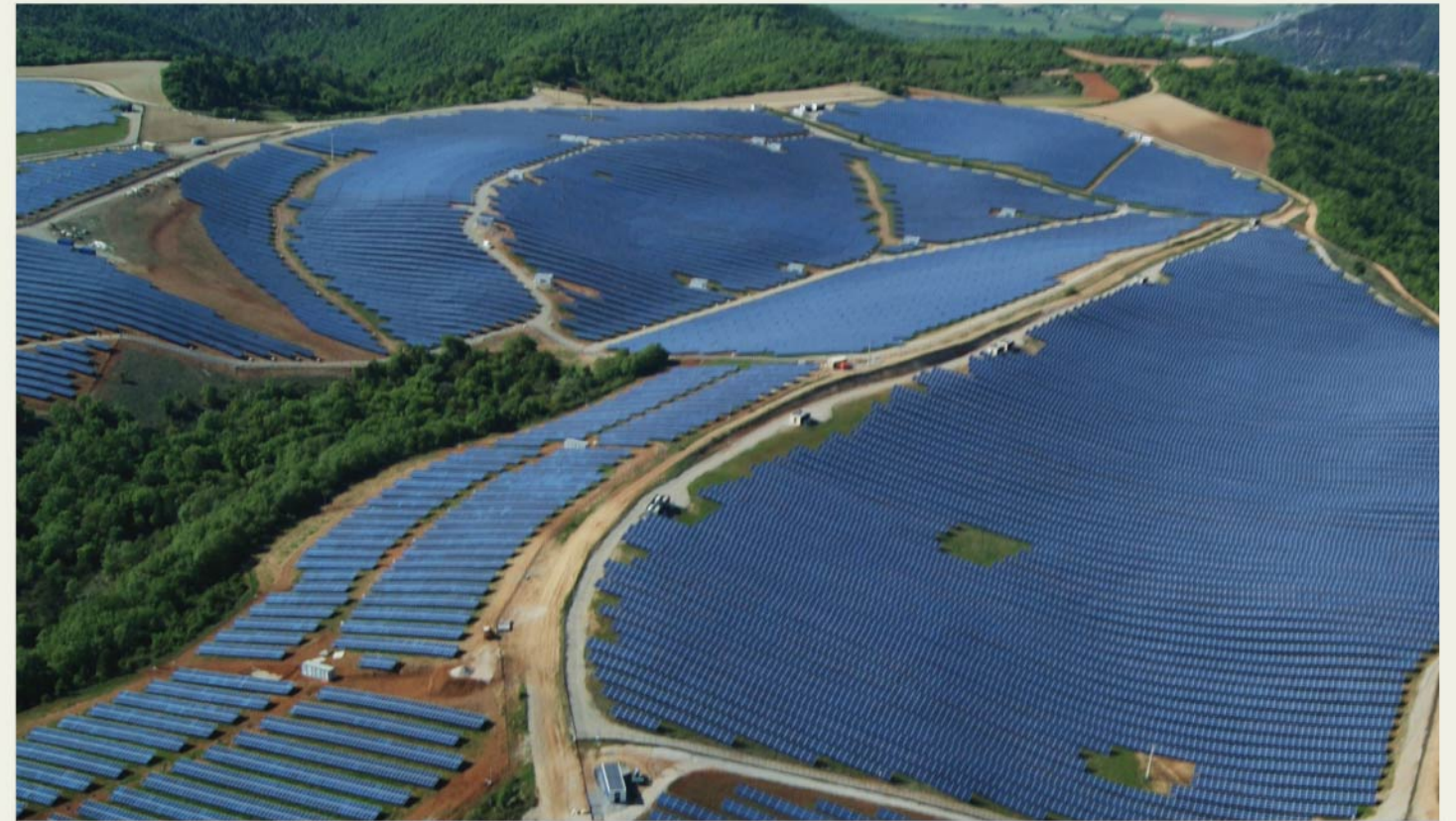
Solar panel fields in Provence, France.
