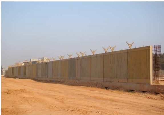
View of Baiyappanahalli Depot
