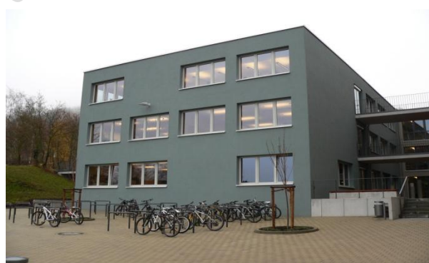
Figure 2: The building of the Lobdeburg School was fully renovated.
