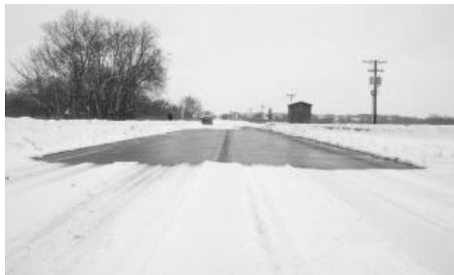
Fig. 7—Roca Bridge deck deicing—February 5, 2004.
