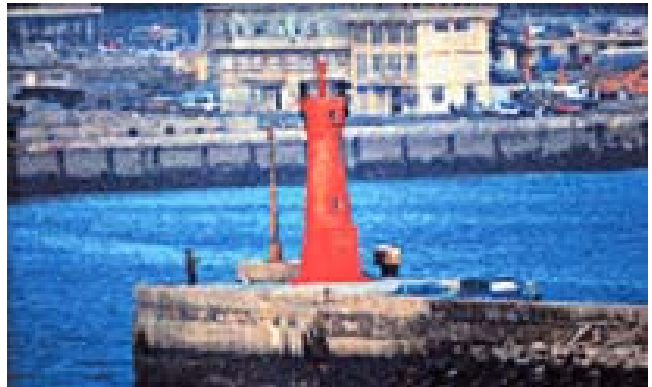
Tai-Chung Inner Breakwater S Light
