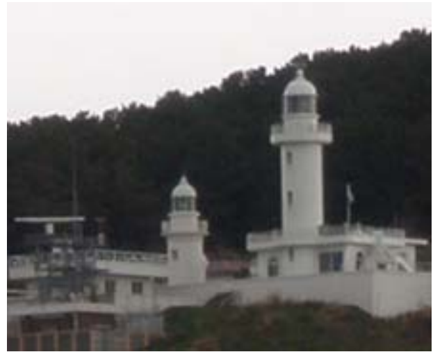
Cheju Hang Traffic Control Center
