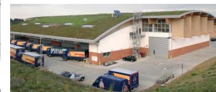
Figure 3.63: Sedum green roofs can provide cost effective biodiversity and improve the outlook of otherwise barren roof spaces
