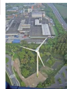
Figure 1.18: Sustainable technology, Reading Green Park
