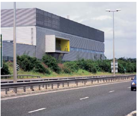
Figure 3.53: The main road frontage of LifeScan Scotland, with innovative yet industrial design, Inverness
