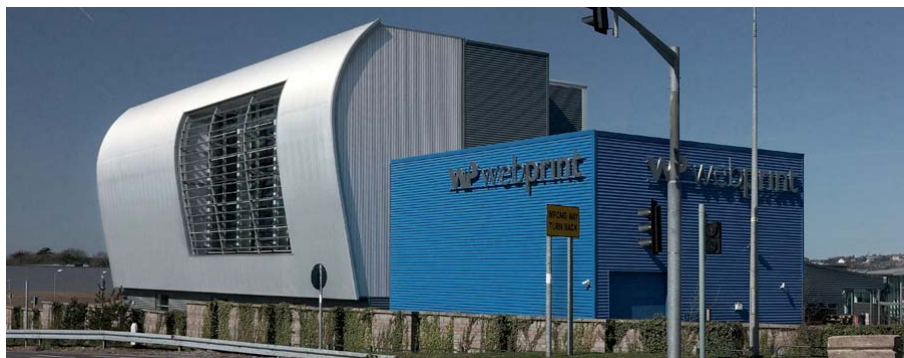
Figure 3.24: Exemplar design for industrial buildings, Thomas Crosbie Holdings, Weblink Manufacturing Facility, Cork
