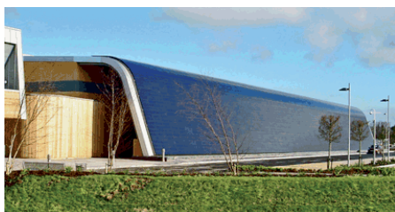
Figure 3.52: Curtain wall photo voltaics as part of the overall design
