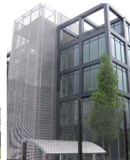
Figure 3.22: Exemplar taller and well designed elements along London Road, Manor Royal
