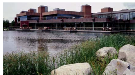
Figure 3.32: Buildings with an active and positive relationship with ecological elements in their context, Marks and Spencer Financial Services, Chester
