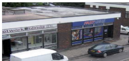
Figure 3.9: Ancillary uses within Manor Royal, Gatwick Road
