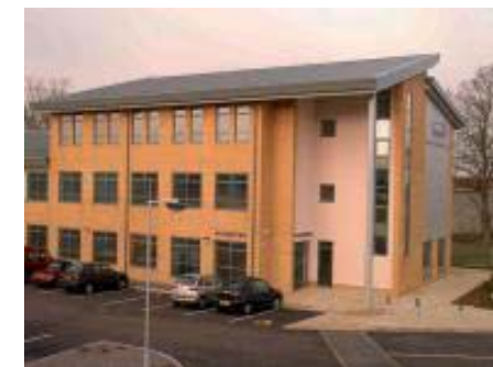
Figure 3.38: Basepoint premises, Manor Royal Fringe
