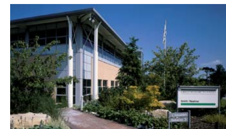
Figure 3.50: Well articulated entrances utilising planting and ground surface treatment to define spaces, Smith and Nephew Building, York Science Park
