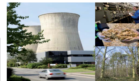
Figure 3.28: Slough Trading Estates energy centre, renewable forests, bio-fuel and control room
