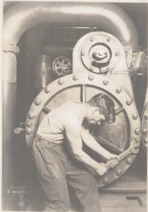
672-- Man at steam pump in a N.Y. power-house An Industrial design By Lewis W. Hine- 1920
