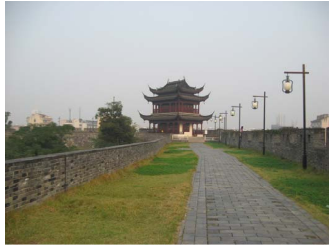
Peripheral Canal: Southeast
