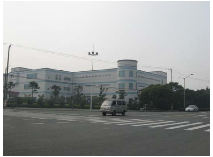
Western Industrial Area
