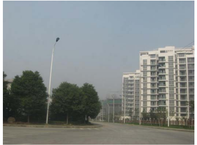
Western Industrial Area
