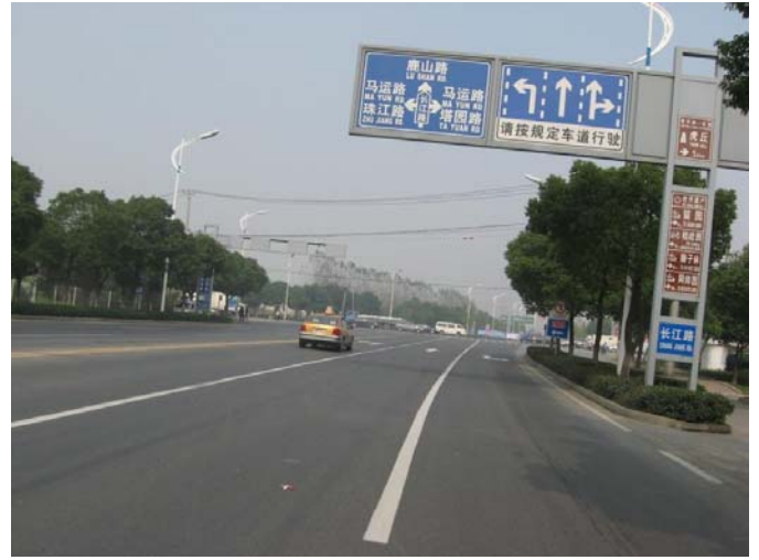
Western Industrial Area
