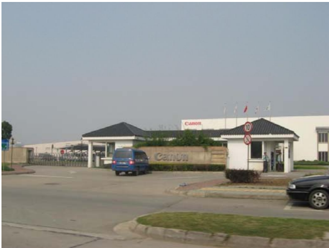
Western Industrial Area
