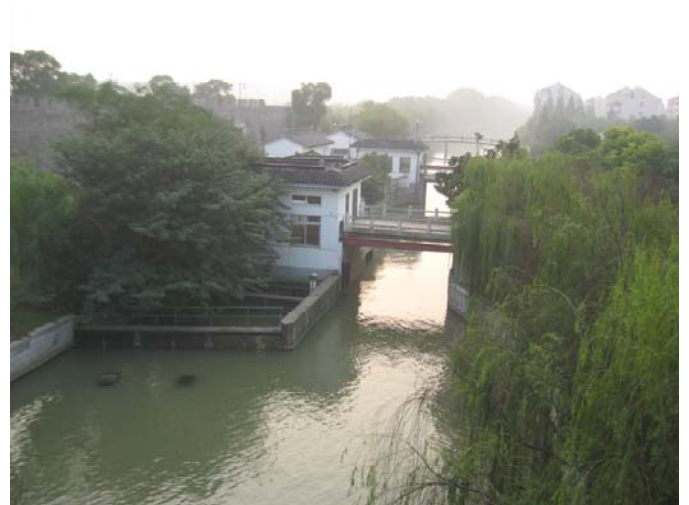
Peripheral Canal: Southeast
