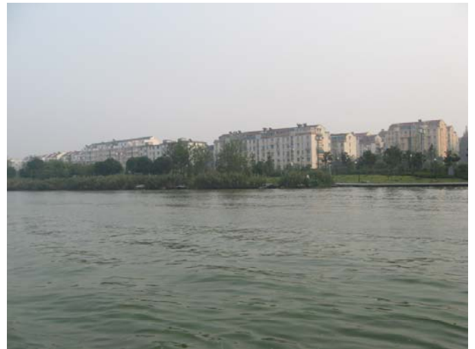
Peripheral Canal: Southeast
