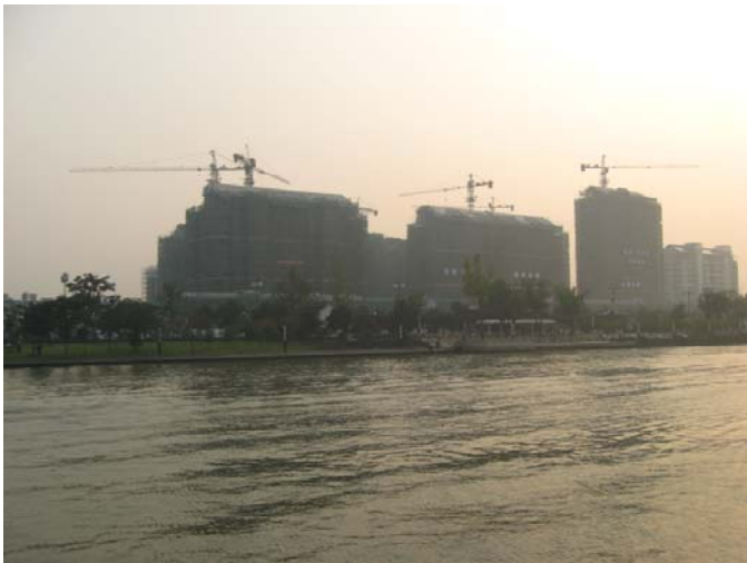
Peripheral Canal: Southeast
