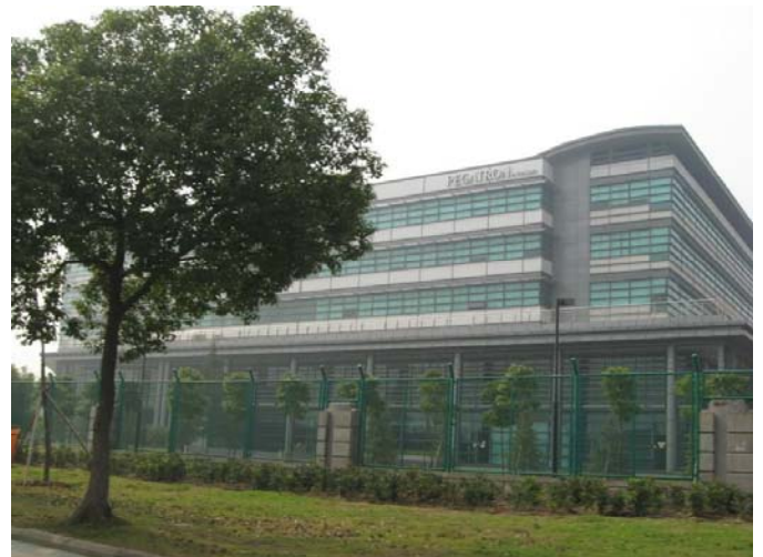
Western Industrial Area
