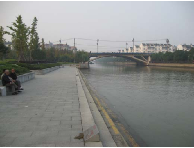
Peripheral Canal: Southeast
