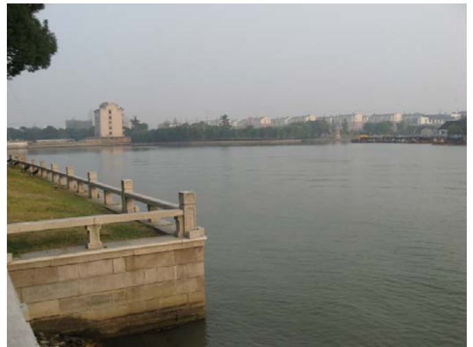
Peripheral Canal: Southeast
