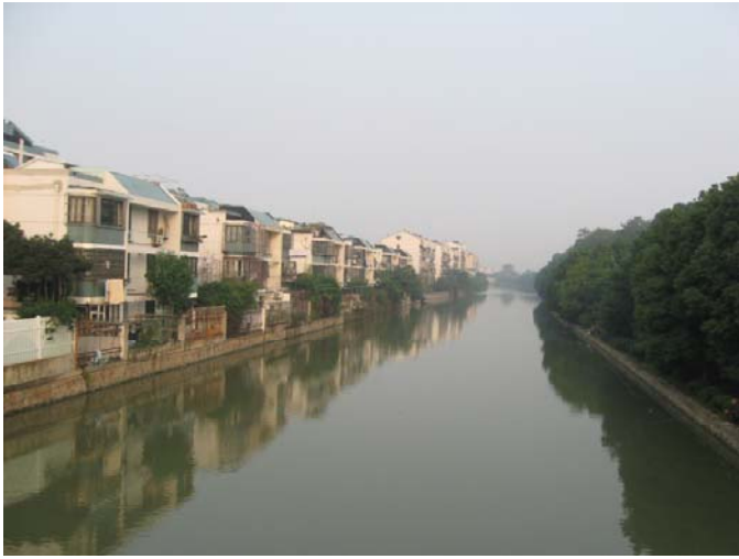
Peripheral Canal: Southeast
