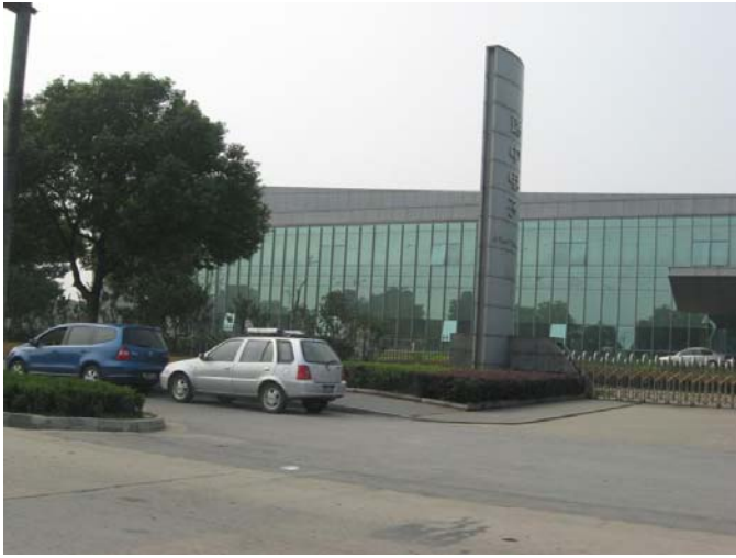
Western Industrial Area
