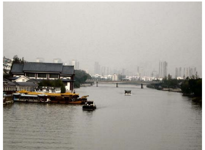
Peripheral Canal: Southeast
