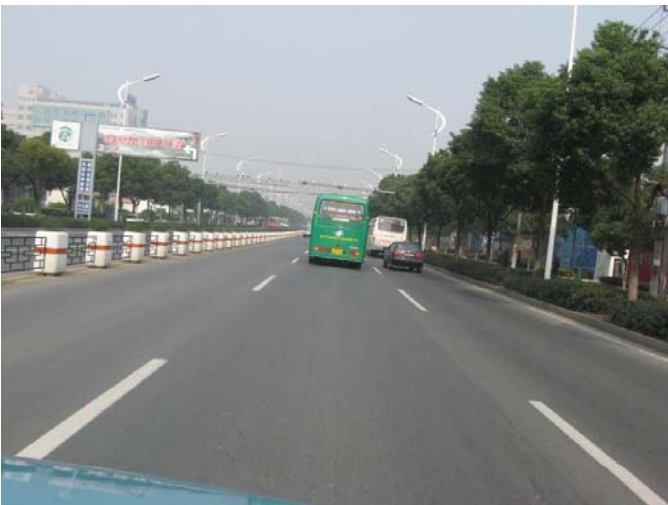
Western Industrial Area
