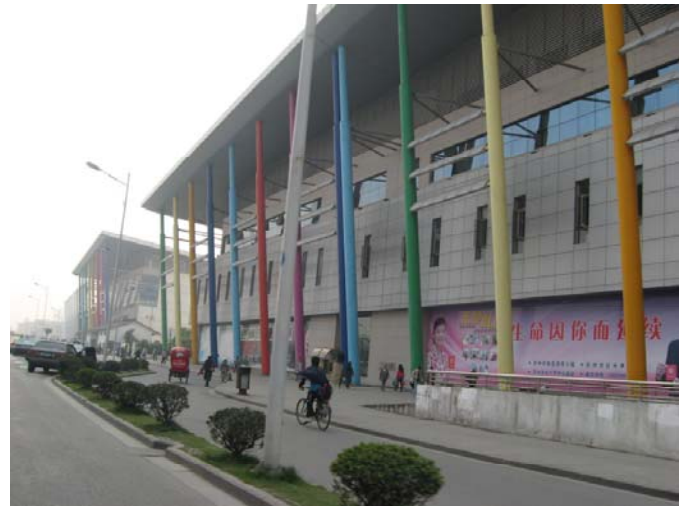
Southern Sector: Shopping Center
