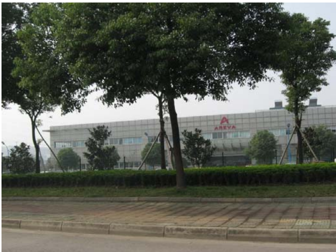
Western Industrial Area
