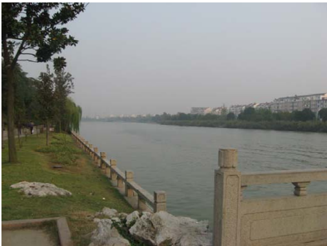
Peripheral Canal: Southeast
