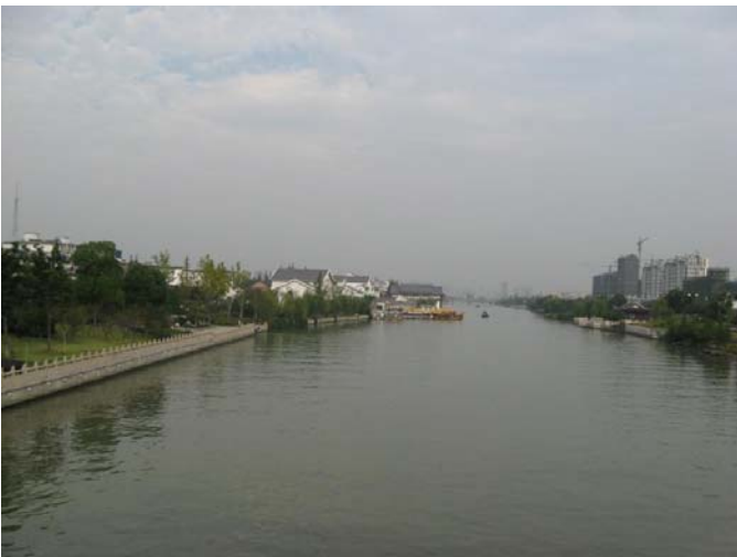
Peripheral Canal: Southeast
