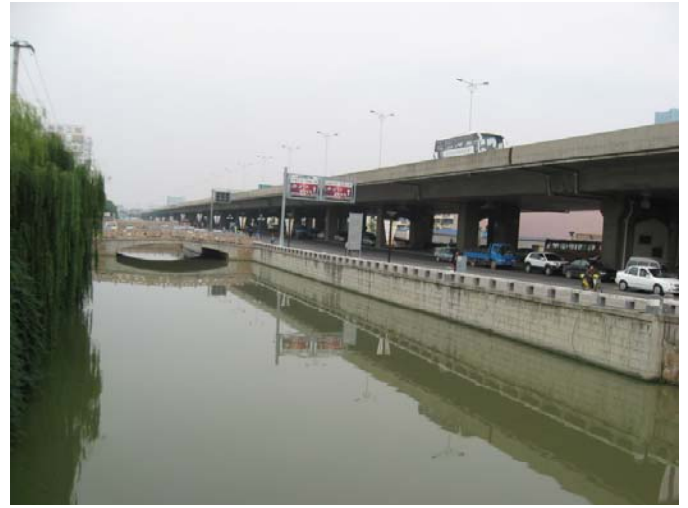
Canal in Western Area
