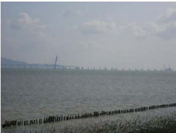
New Hong Kong-Shenzhen Bridge
