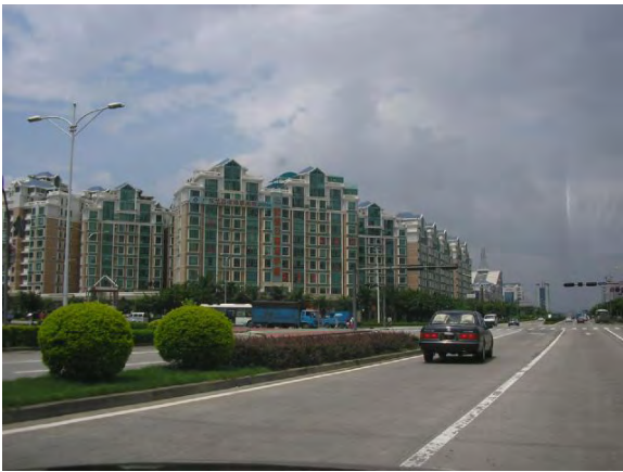
Longgang (Exurb of Shenzhen)
