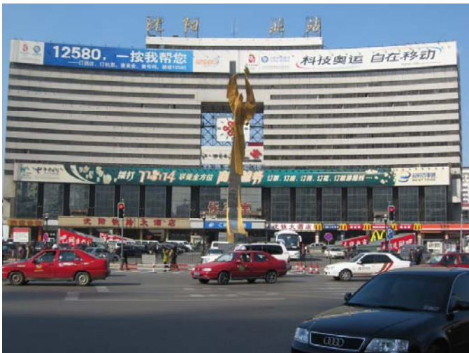
North Railway Station
