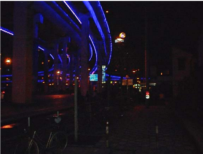
Central Motorway Interchange: Night 5
