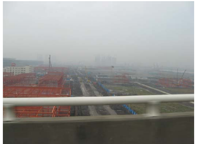
Construction at 2010 Expo Site
