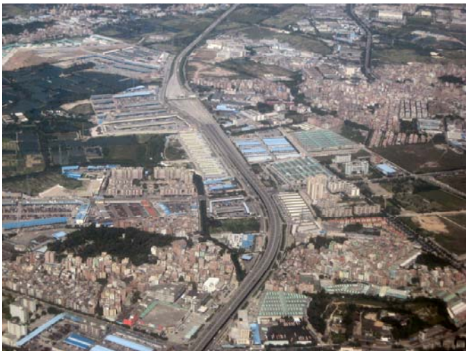
Guangzhou (North): Toll Plaza on Expressway
