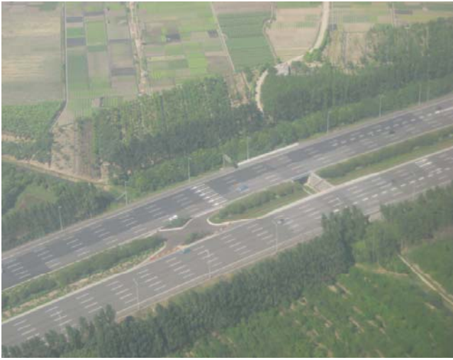
Guangzhou (North): 12 Lane Expressway
