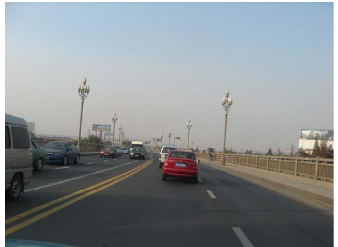
Yangtze River Bridge
