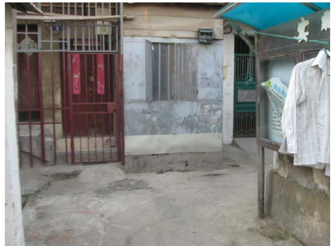
Inside the South Wall: Substandard Housing 162
