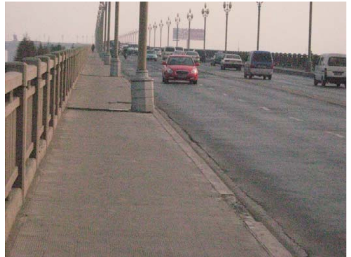
Yangtze River Bridge
