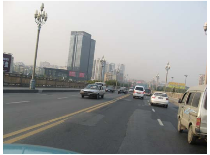
Yangtze River Bridge
