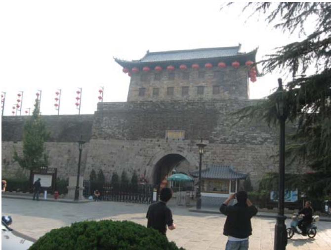
Inside the South Wall
