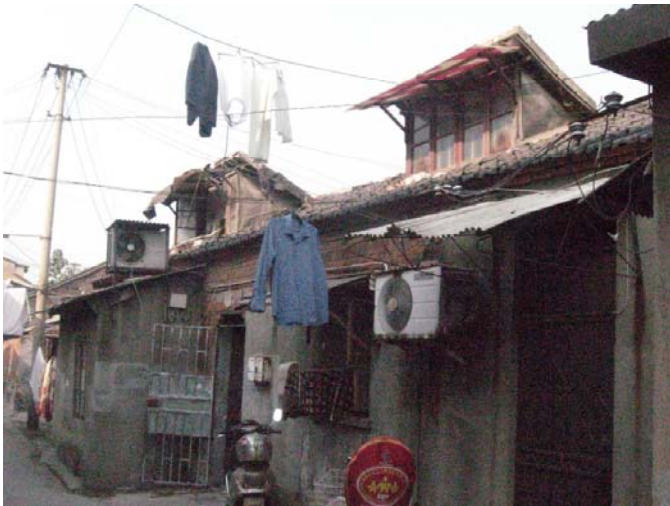
Inside the South Wall: Substandard Housing
