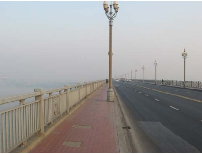
Yangtze River Bridge
