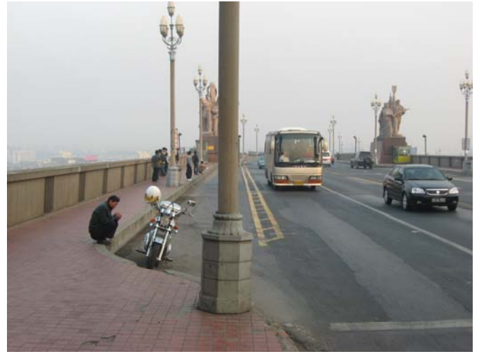
Yangtze River Bridge
