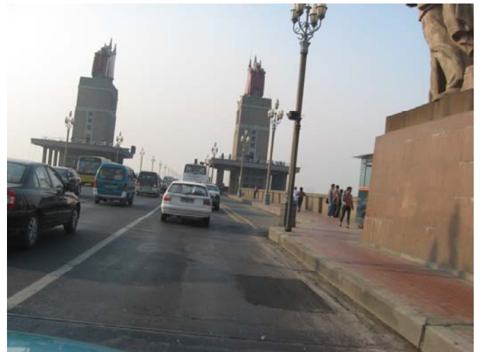
Yangtze River Bridge
