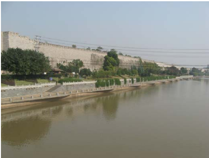
South Wall & Moat
