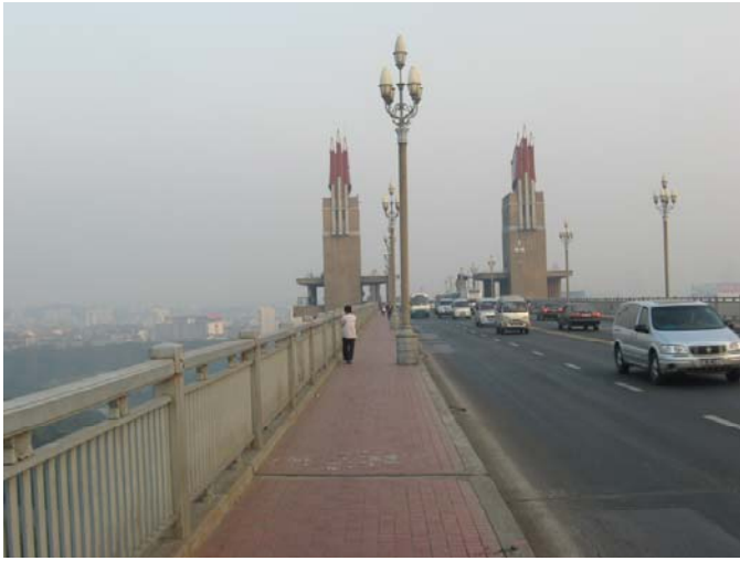
Yangtze River Bridge
