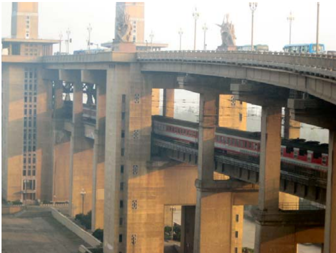
Yangtze River Bridge: Passenger Train on Lower Deck
