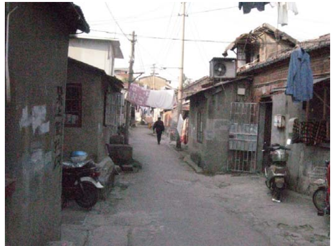
Inside the South Wall: Substandard Housing
