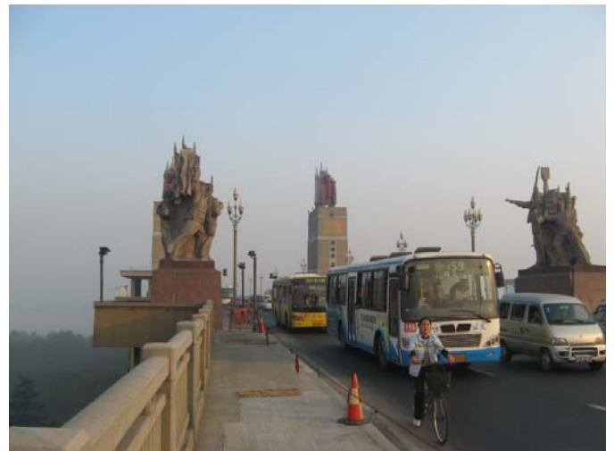
Yangtze River Bridge
