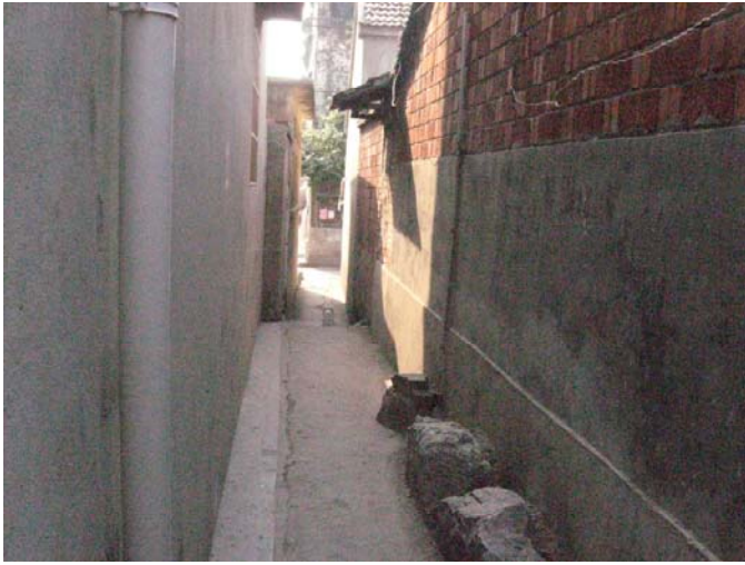
Inside the South Wall: Substandard Housing 157
