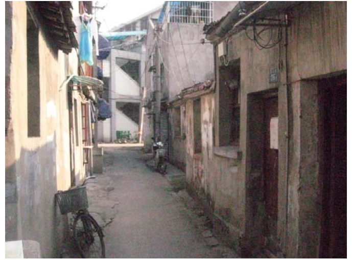
Inside the South Wall: Substandard Housing
