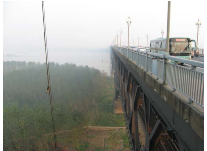
Yangtze River Bridge
