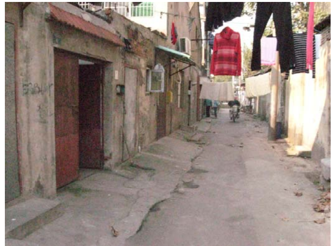
Inside the South Wall: Substandard Housing 166
