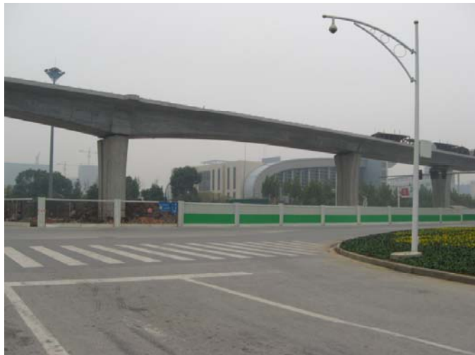
Eastern Area: Metro Construction
