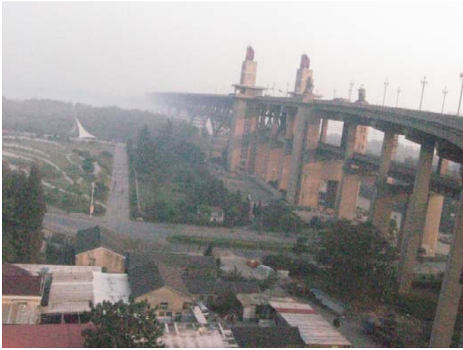
Yangtze River Bridge
