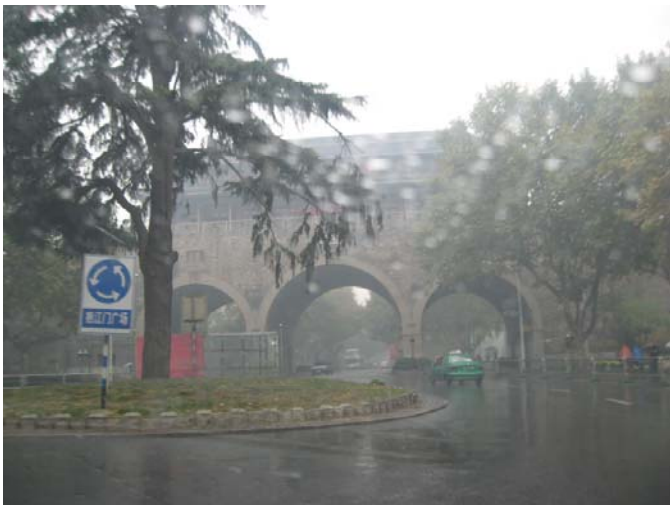
Western Area: Y Chang Men Gate
