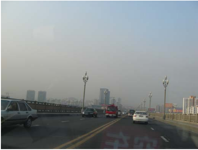
Yangtze River Bridge
