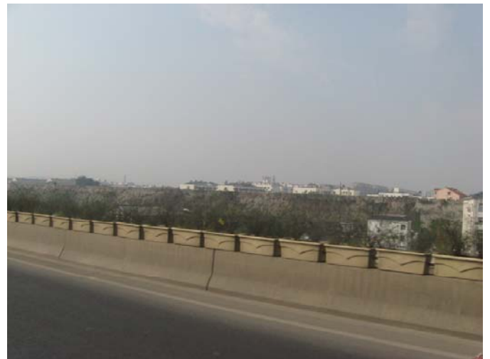
South Wall from Freeway
