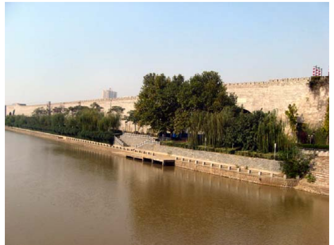
South Wall & Moat
