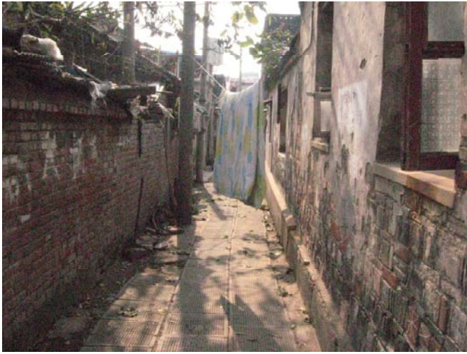
Inside the South Wall: Substandard Housing
