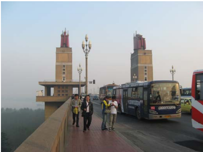
Yangtze River Bridge
