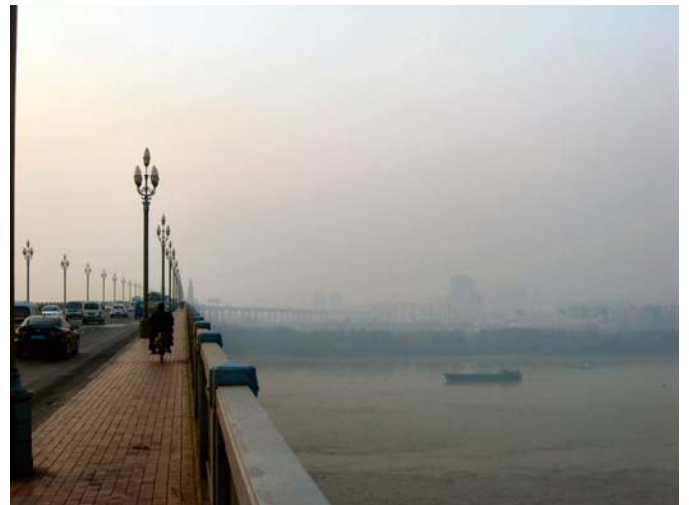
Yangtze River Bridge
