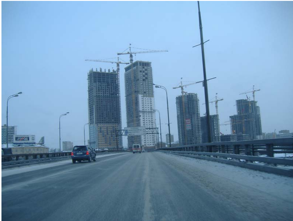
Residential Construction: Moscow
