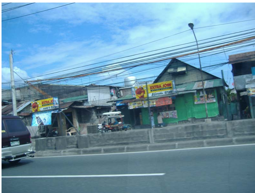
Development Along South Superhighway
