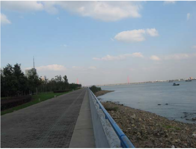
Qiantang River Floodwall
