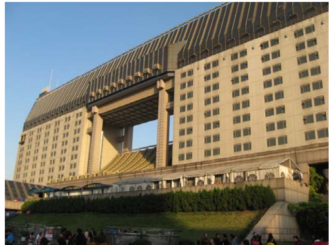
Hangzhou Railway Station
