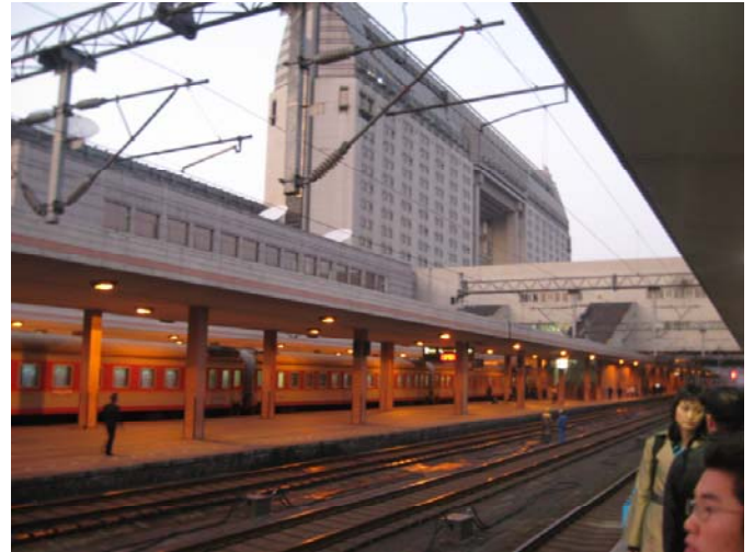
Hangzhou Railway Station
