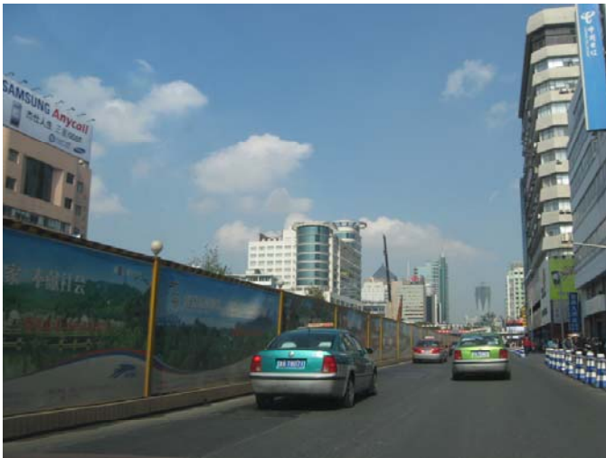
Historic Core: Metro Construction
