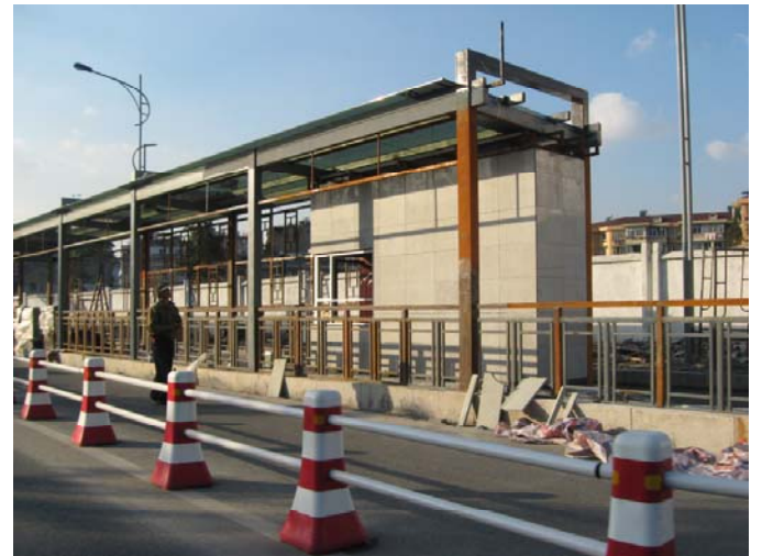
Bus Rapid Transit Construction
