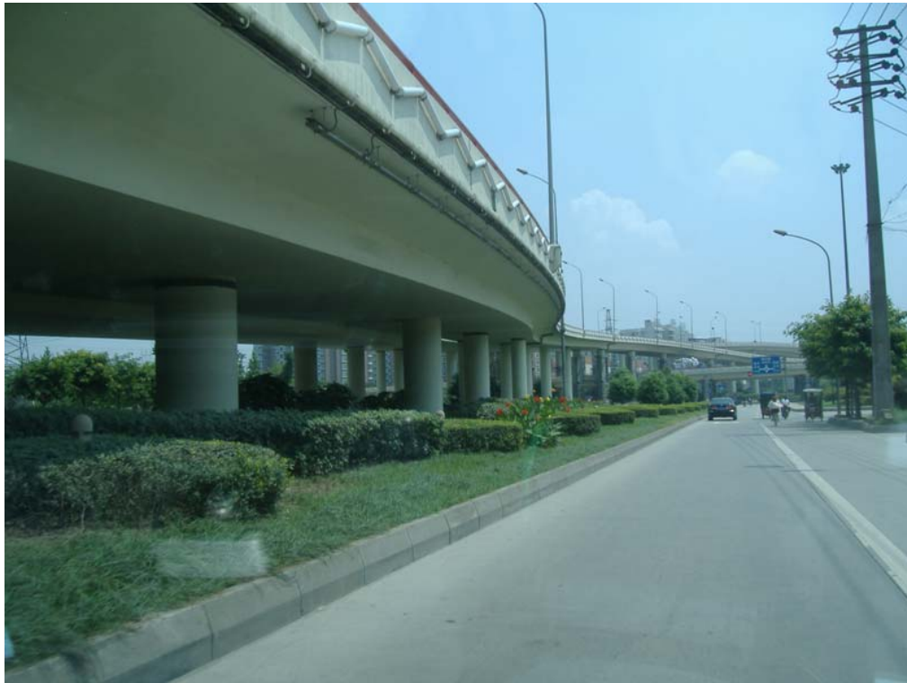
Chengdu: Western Development Area
