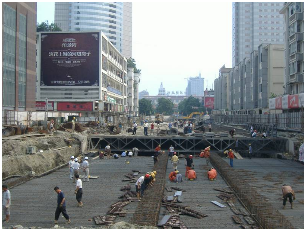
Chengdu: CBD (Metro Construction)
