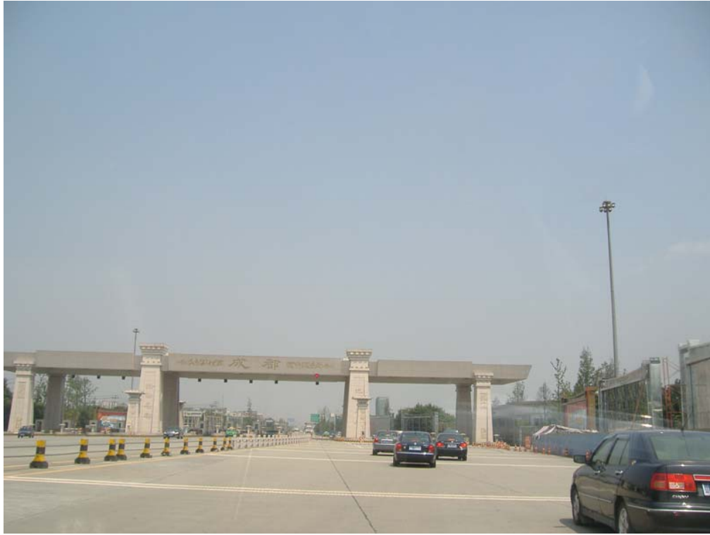
Chengdu Airport Expressway Toll Booth
